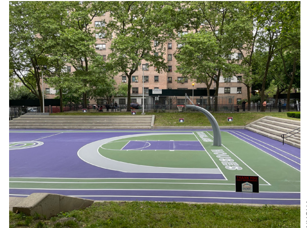
New York City's cloudburst infrastructure.
