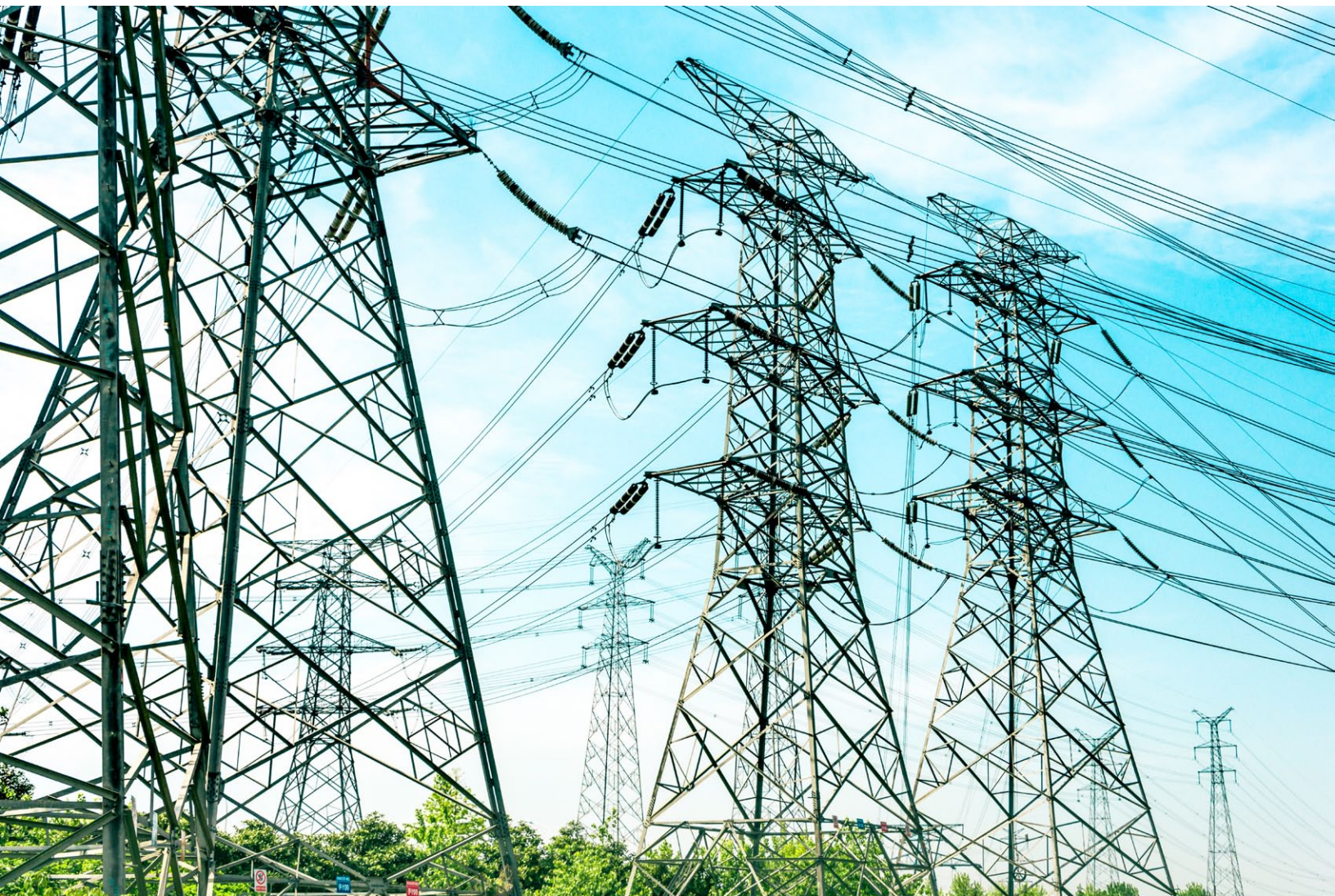
Aboveground utility wires are more likely to be damaged by climate disasters, like storms and high-wind events.
