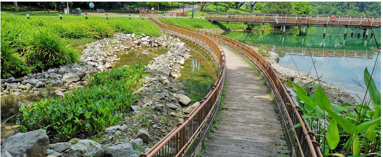
A vegetated gravel swale in MacRitchie Reservoir Park, Singapore, channels rainwater into the drainage network and filters pollutants to enhance the city's water quality.
