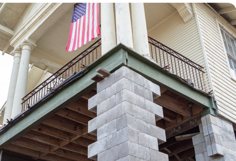
Elevating buildings above the floodplain is feasible for some smaller, detached structures (left); others may need flood barriers (right).
