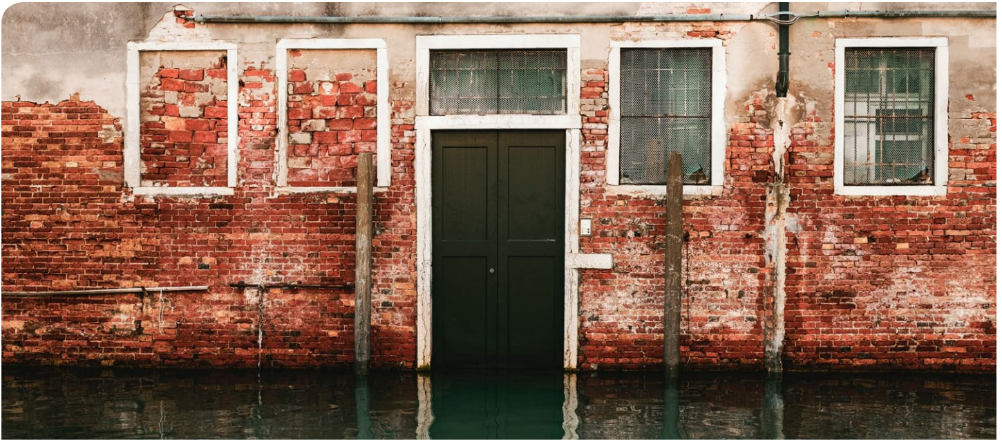
Flooding poses unique threats to historic buildings.
