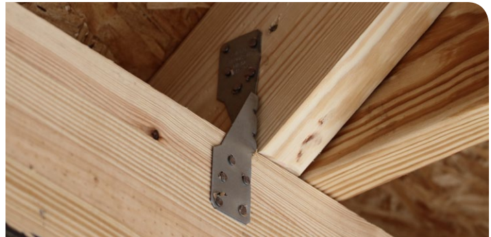
Clips help secure roofs to walls, increasing resistance to winds and earthquakes.
