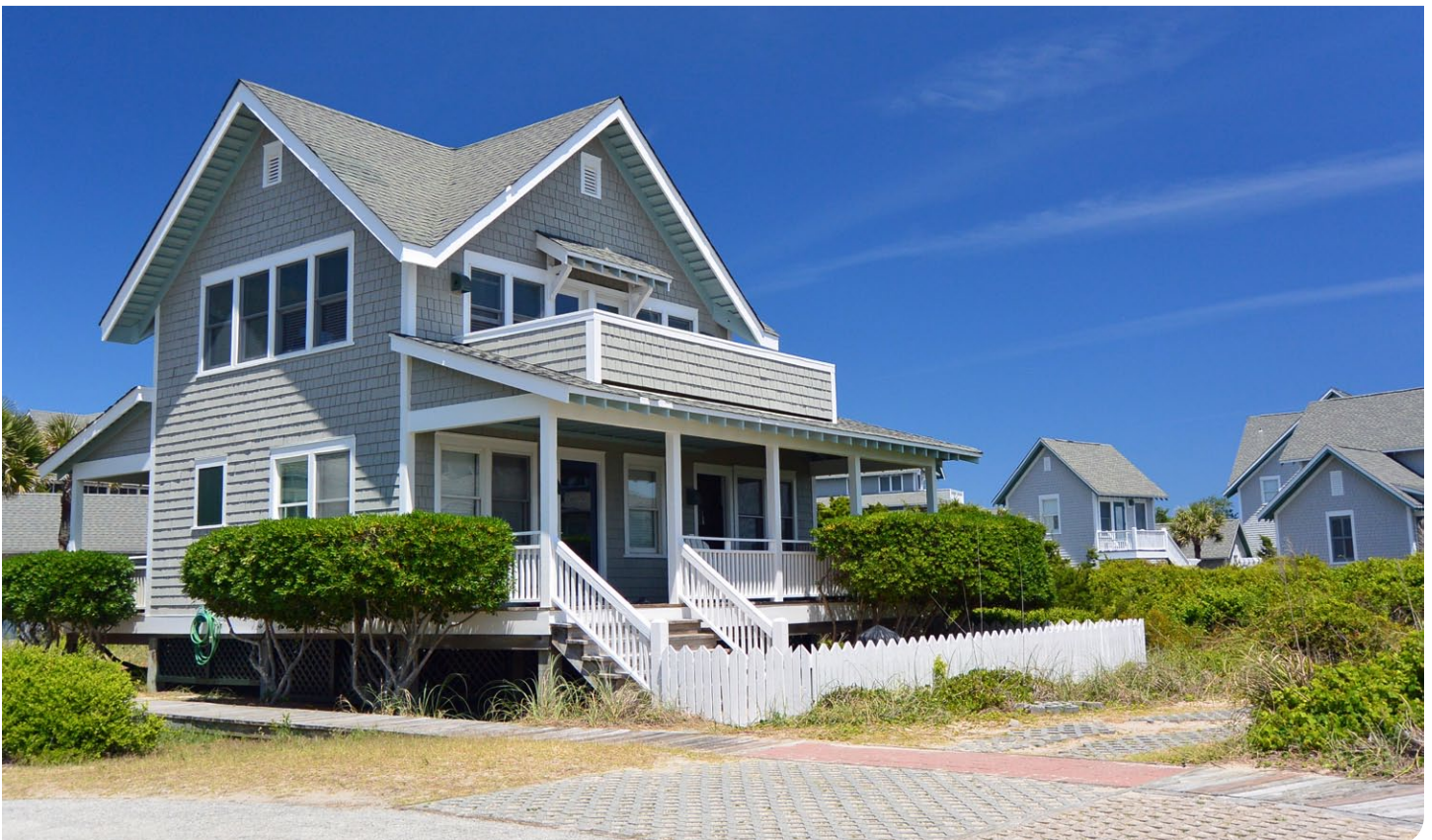
Flexible zoning rules can allow buildings to exceed height limits if they need to be elevated.
