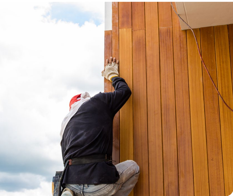
Fiber cement siding can be made to resemble wood and provide fire resistance (left); metal or tile will also protect roofs from ignition (right).
