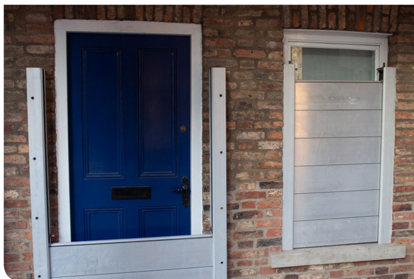
Elevating buildings above the floodplain is feasible for some smaller, detached structures (left); others may need flood barriers (right).
