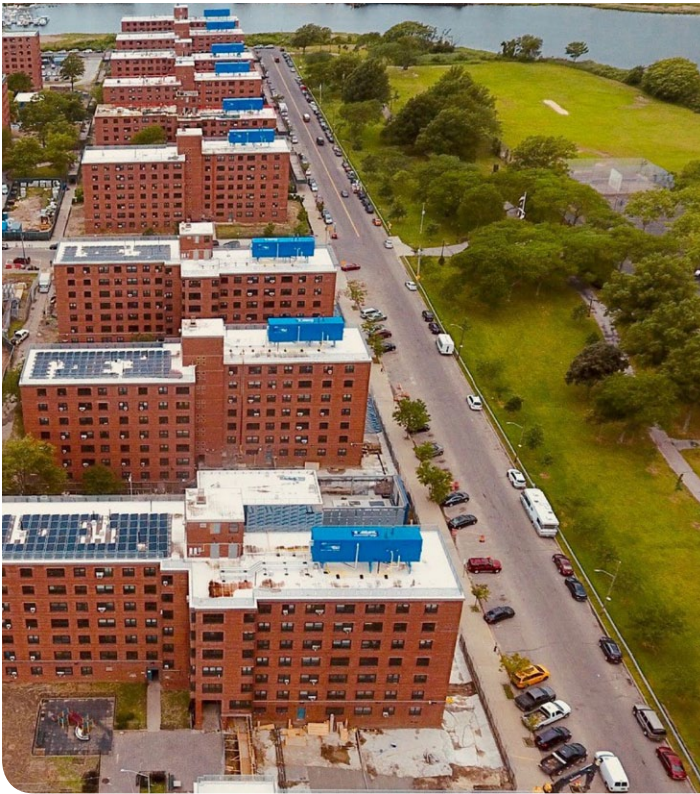
Relocated mechanical equipment (blue) accompanies new solar panels. ( Flood Resilience at NYCHA )
