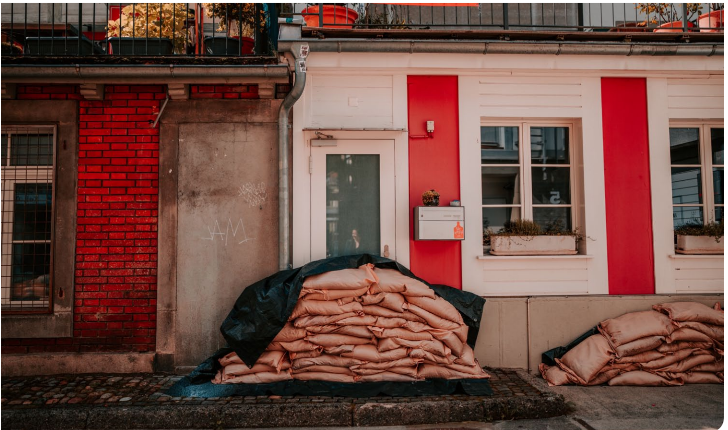
In a pinch, sandbags can be used as a low-tech “temporary retrofit” option and stepping stone to enhanced floodproofing.
