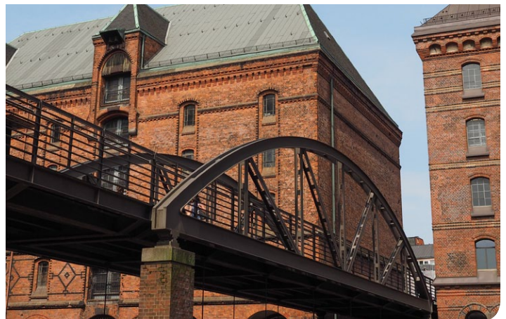
Access to historic buildings during flood events is maintained via connected, raised walkways.
