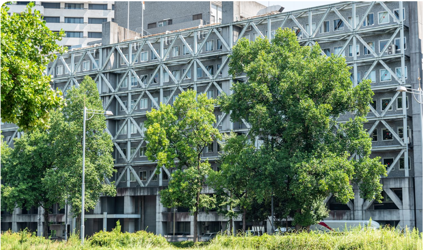
Exterior braces can help reinforce buildings against seismic risks.
