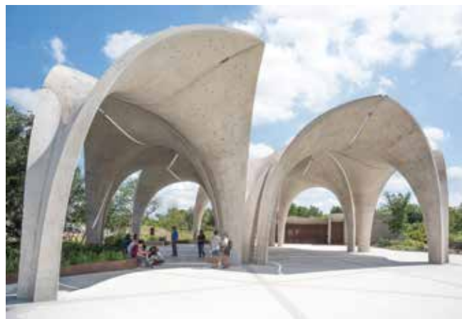
The pavilions at Confluence Park, San Antonio.
