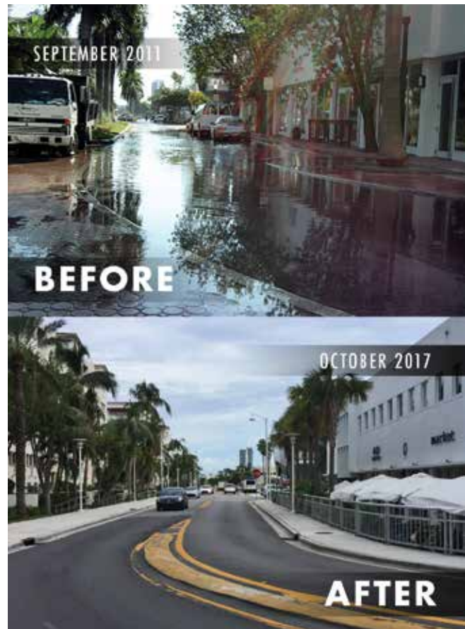
Miami Beach street flooding on 20th Street, before and after stormwater management plan work.
