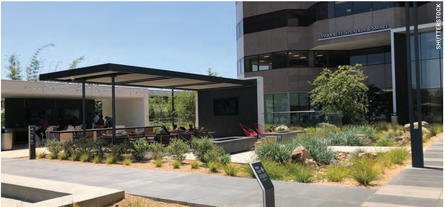
Signage can be used to inform visitors, tenants, and staff about water conservation efforts, like these signs for drought-tolerant landscaping.
