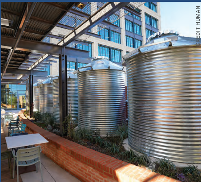
A combination of rainwater capture, storage, and reuse systems make the Credit Human headquarters one of the most water-conscious developments in Texas.
