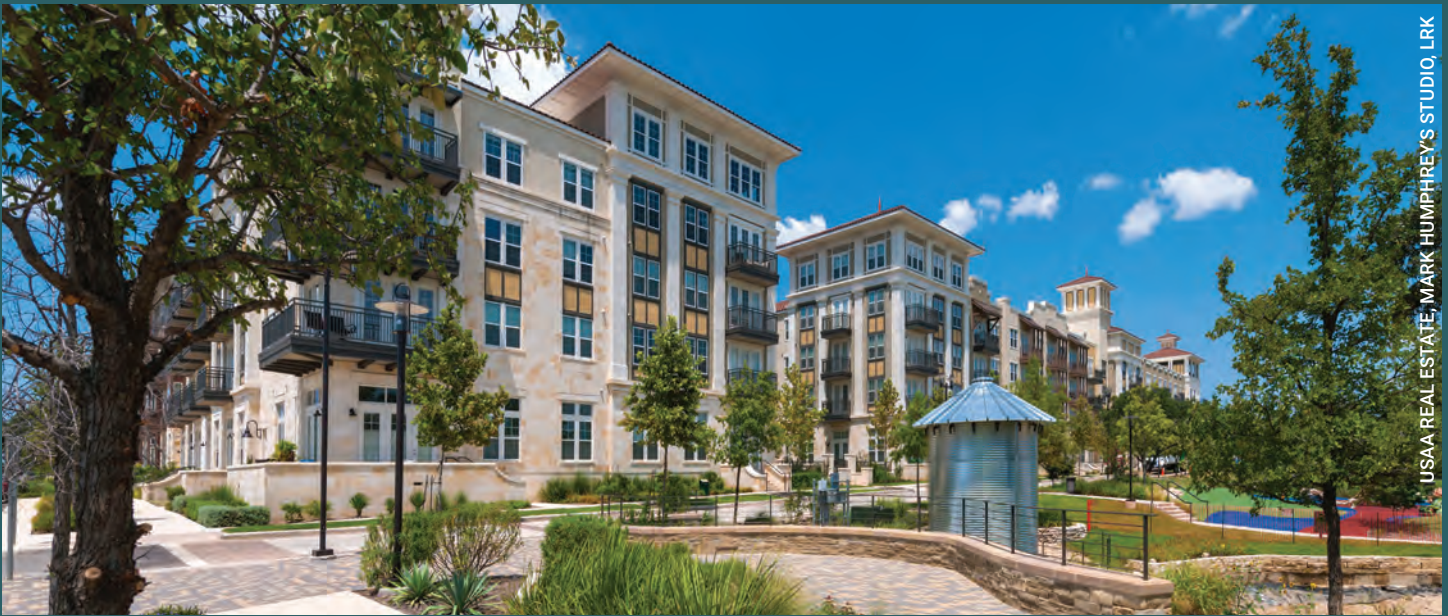
Drought-tolerant plants and a cistern that captures rain and air-conditioning condensate for irrigation help protect the park amenity at the Residences at La Cantera from drought.
