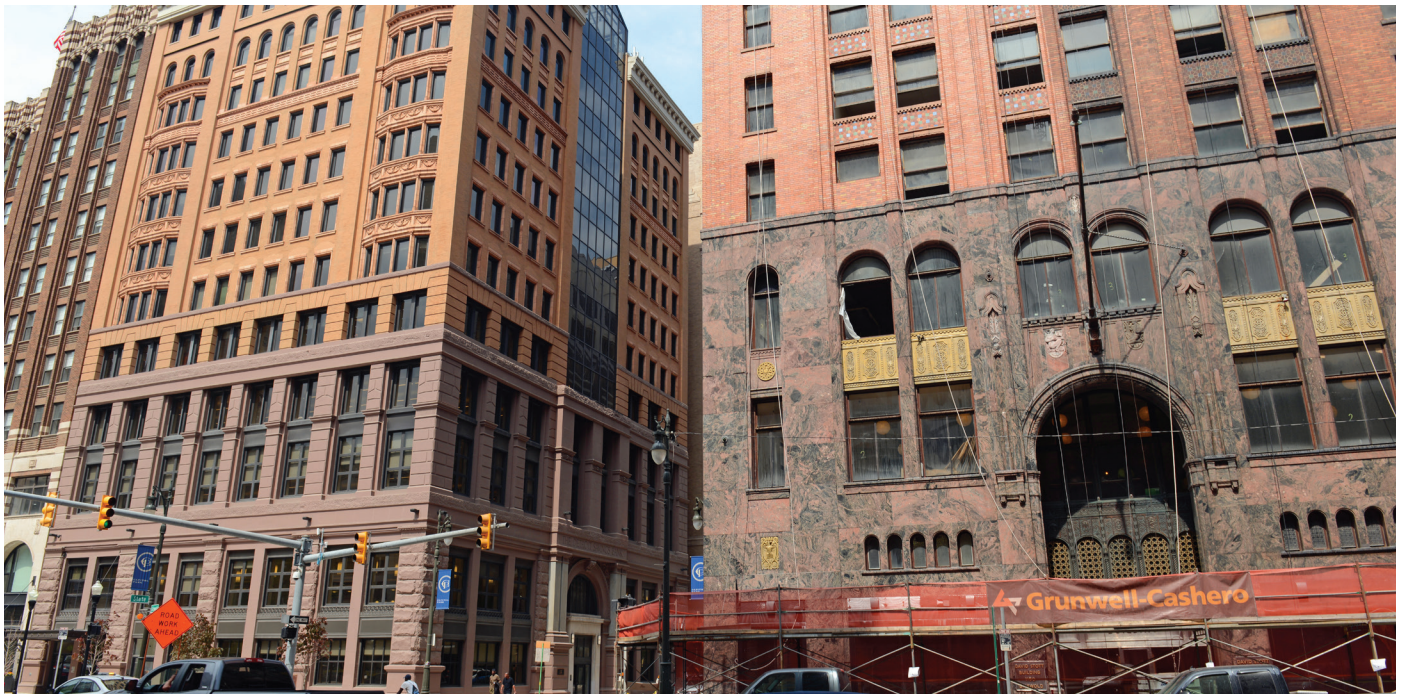
A historic building undergoing rehab.
