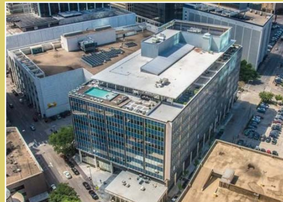
Top: View from street Above: Bird's-eye view after conversion Credit: HRI Properties LLC
