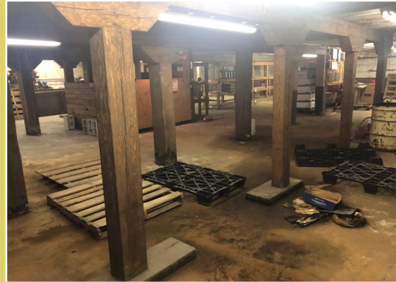
Top: Interior during conversion Credit: Gavin Design Group
