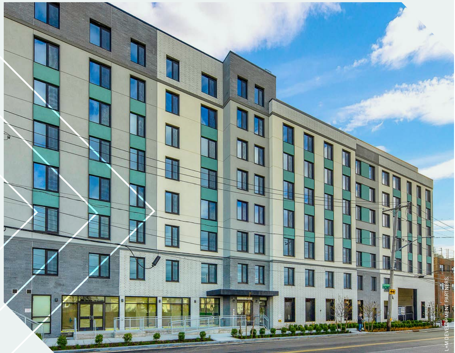
Beach Green Dunes II features an efficient envelope and solar and geothermal energy.
