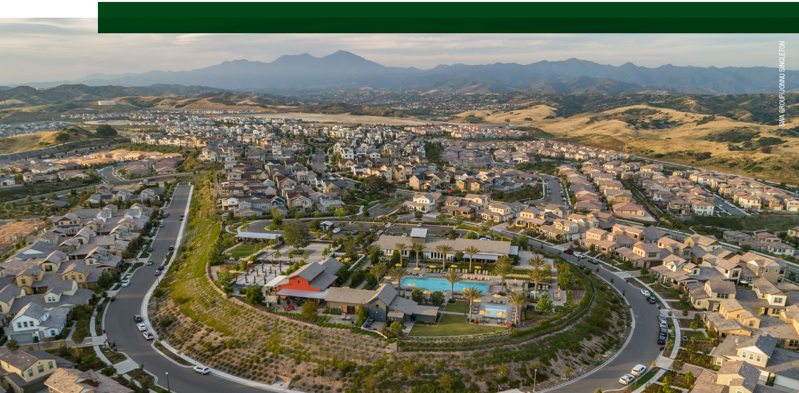
Rancho Mission Viejo, a large residential development in California. The project combines a fire master plan, conservation of open space, building guidelines such as noncombustible material requirements, and strict landscaping and defensible space protocols to reduce risk from wildfire. Learn more at ULI's Developing Urban Resilience site.
