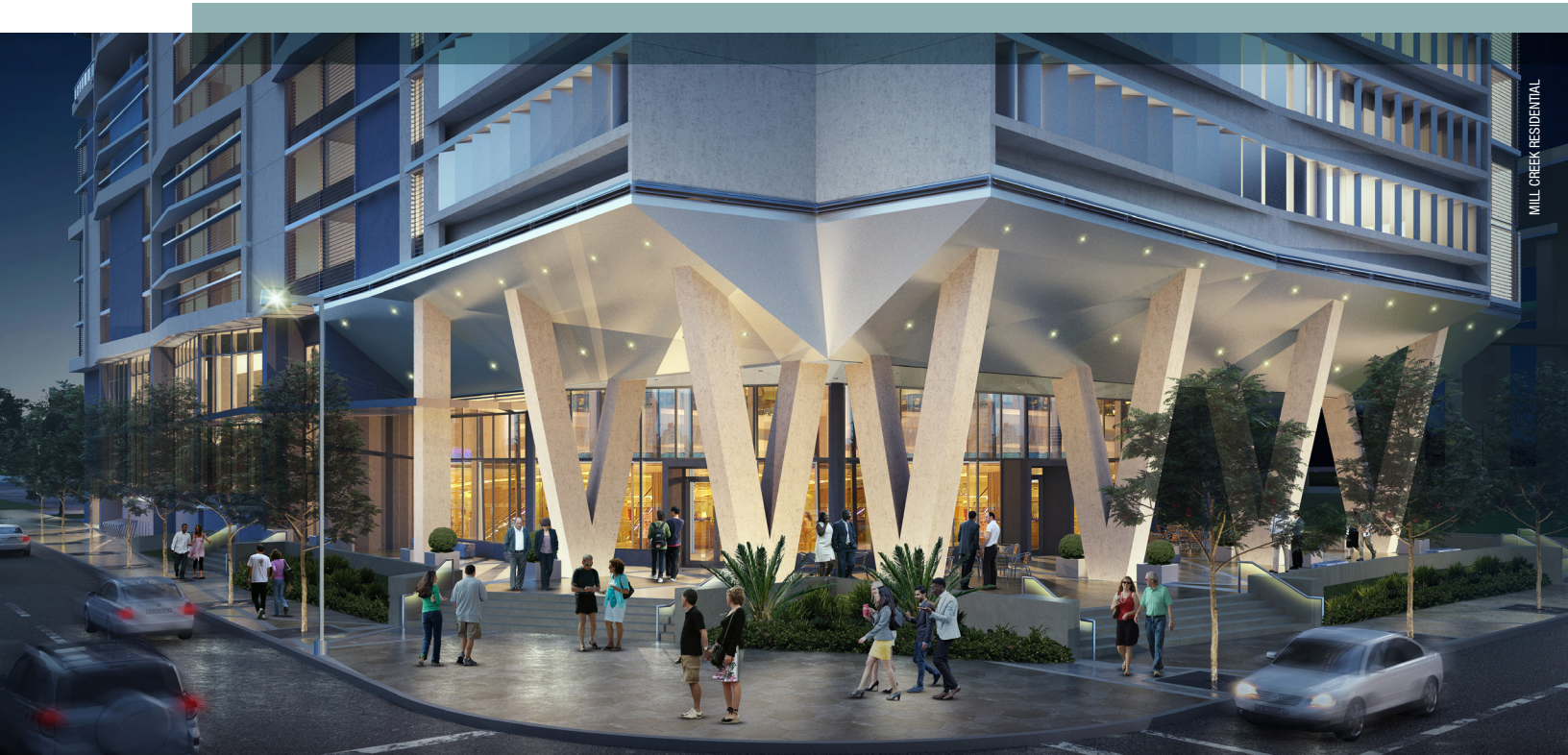
Modera Riverside in Miami, Florida, by Mill Creek Residential, uses a raised ground-floor platform to reduce flood impacts, and high ceilings on the ground floor allow the interior floor elevation to be raised in the future to keep up with potential raising of municipal infrastructure and streets.
