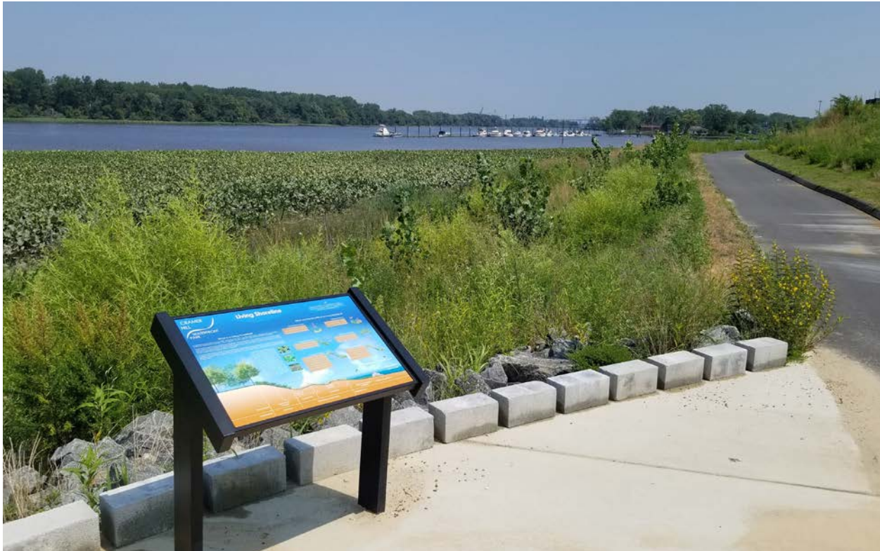
Over 3,000 feet (914 m) of shoreline was regraded and stabilized to create a buffer against riverine flooding.
