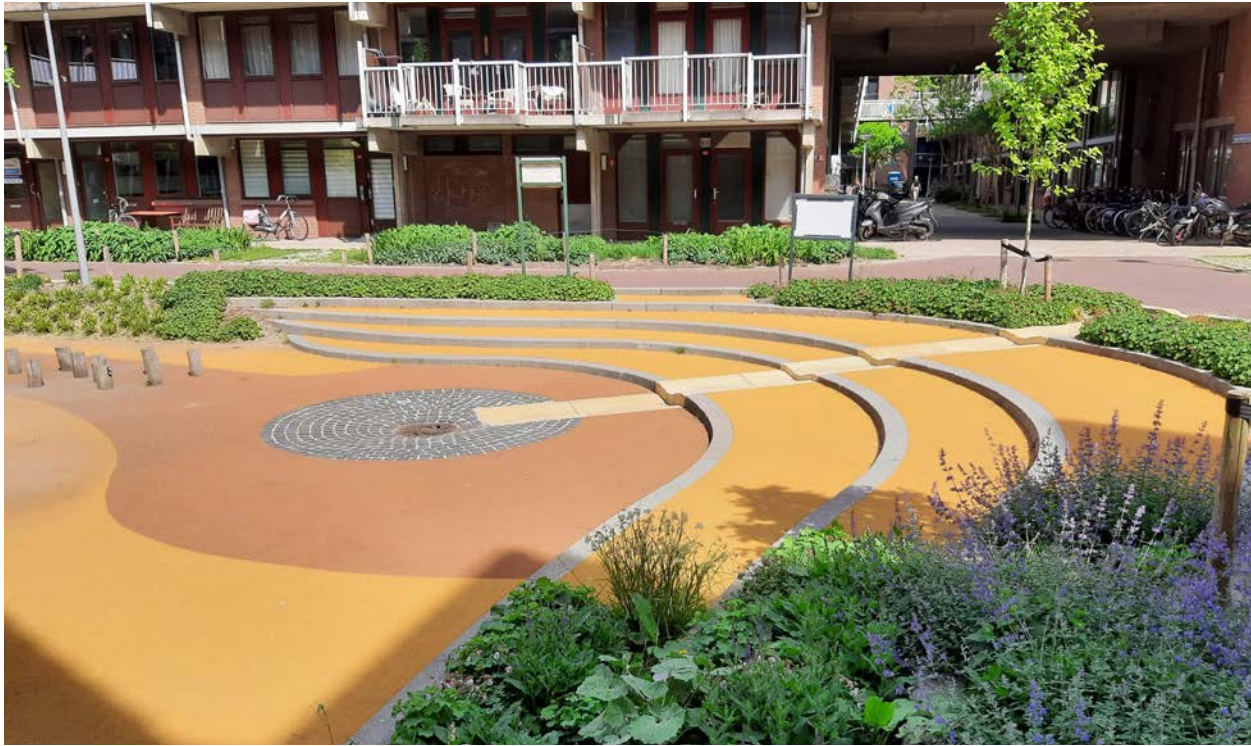
At Heliport, native plants capture and filter stormwater while a series of cascading steps direct runoff to a central storm drain.
