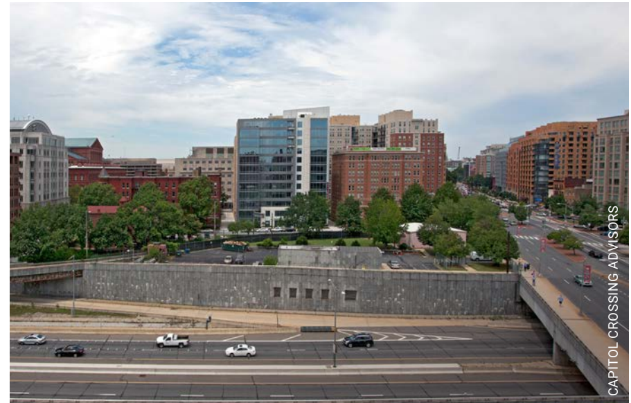
Capitol Crossing site before decking over I-395.
