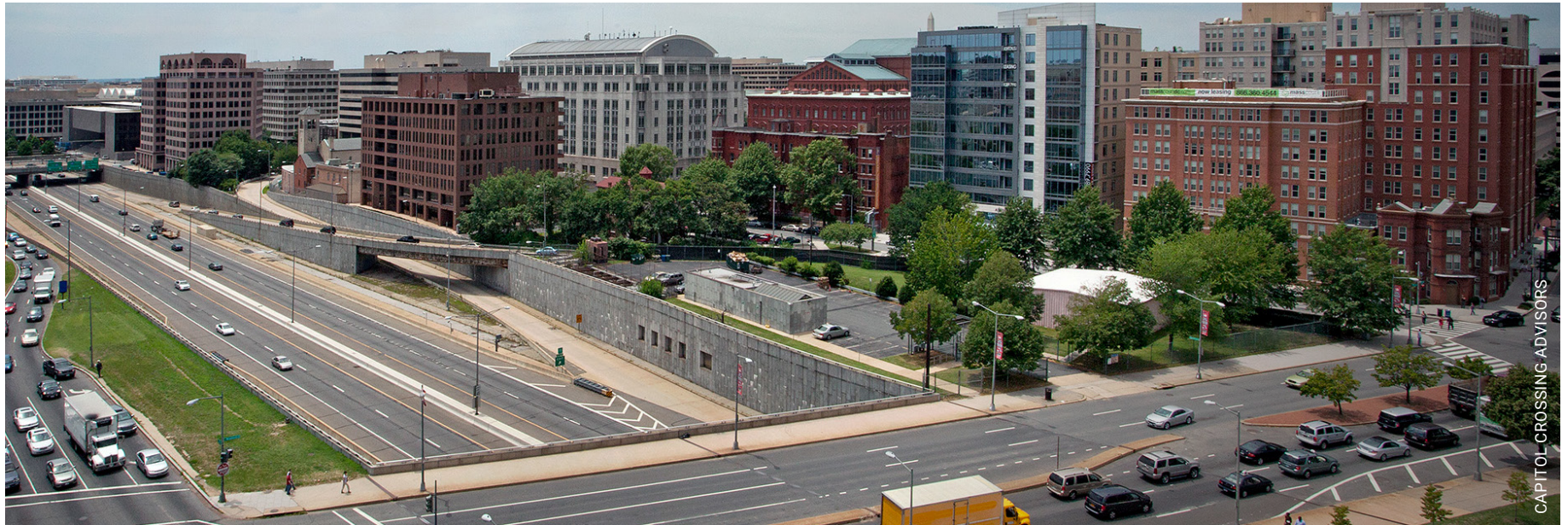
Capitol Crossing site before decking over I-395.
