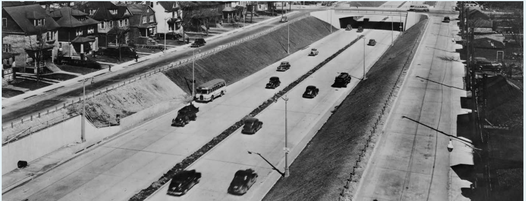
Built in 1941–1942, the Davison Freeway in Detroit and Highland Park, Michigan, was one of the first depressed urban freeways in the United States; construction required that dozens of homes be moved or demolished.
