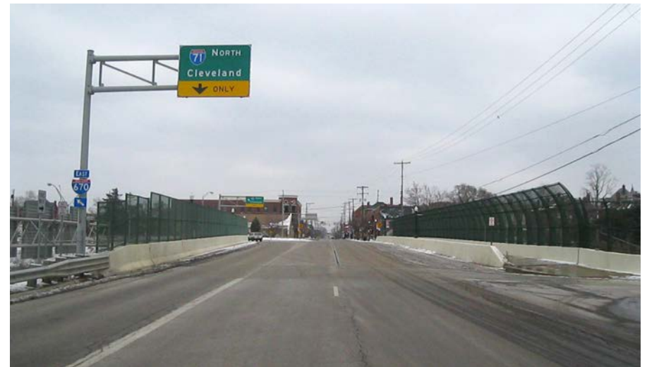
Long Street Bridge before transformation.
