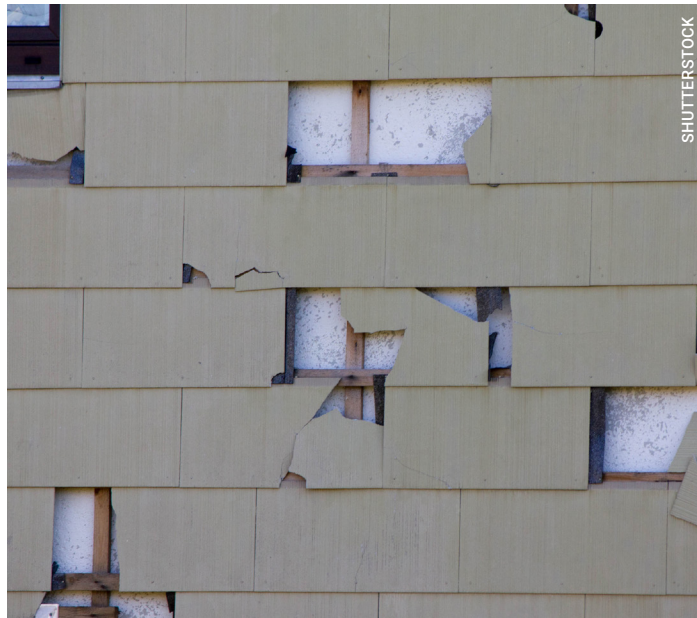
Hail, though not restricted to episodes of extreme cold, can cause millions of dollars of damage to roofs and facades.
