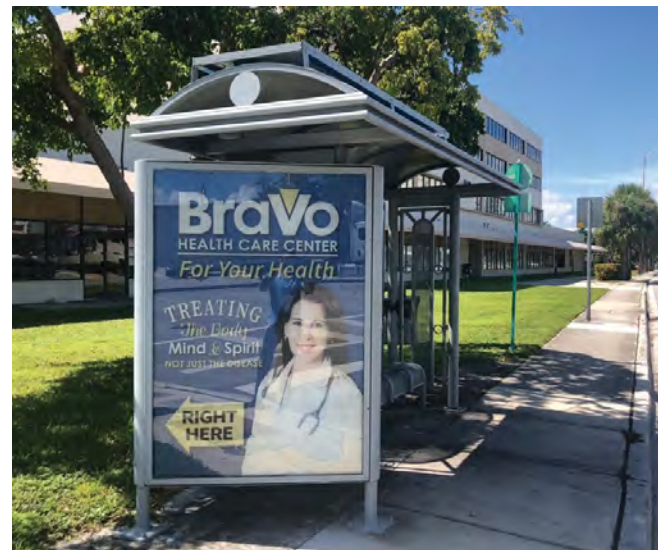
Existing bus shelter
