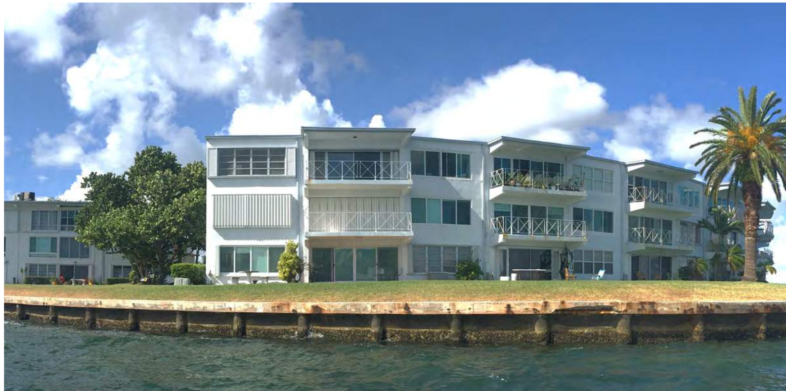
Current Condition of Seawalls
