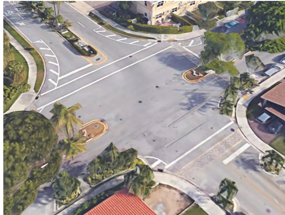
Existing intersection at N. Treasure Drive and Hispanola Dr.
