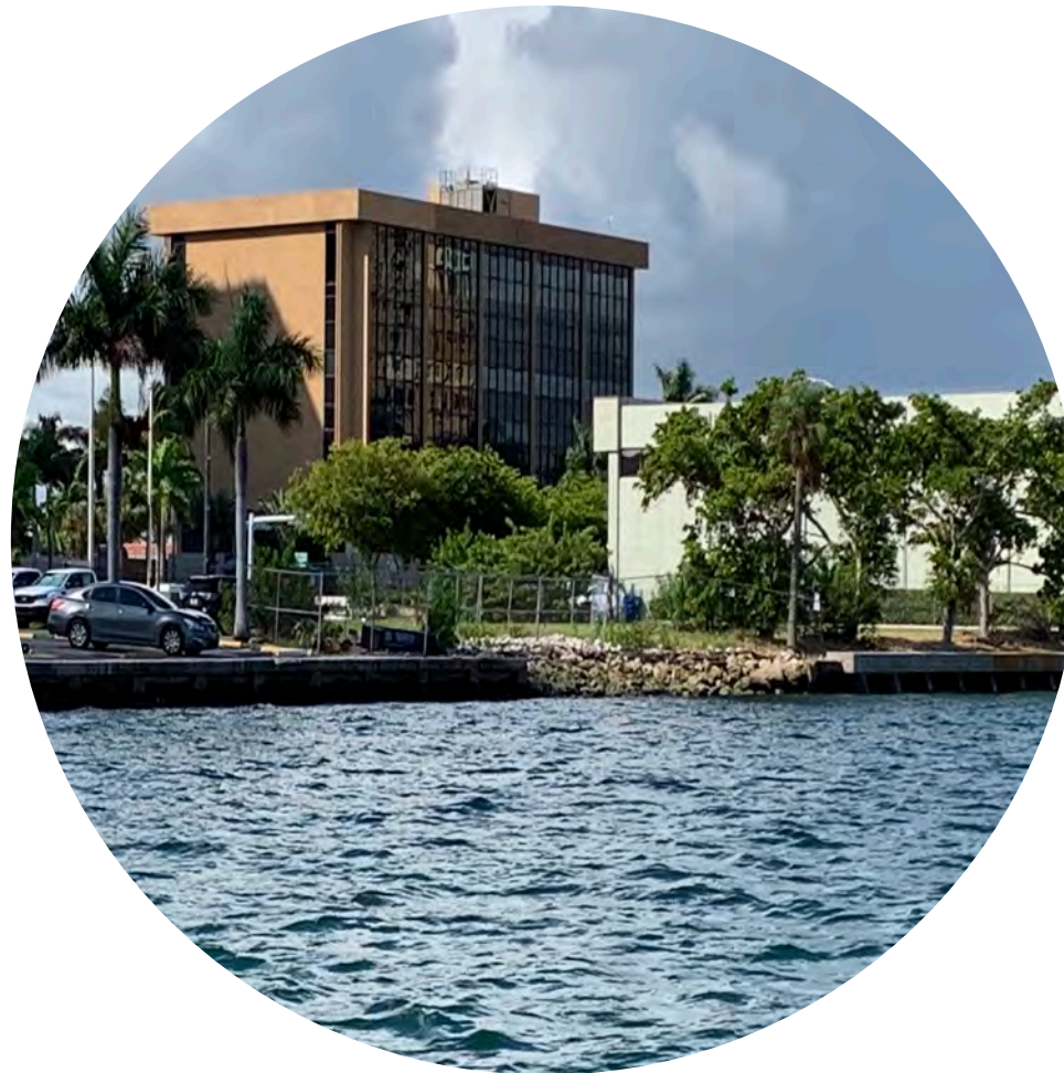
Seawalls at different states of repair
