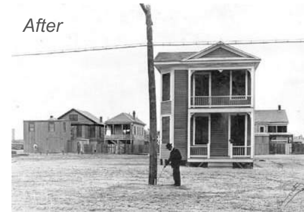
In the before photo, a surviving house has already been raised to the new elevation. A man points to this elevation painted on the utility pole high above his head. In the after photo, the ground level has been filled in below, creating a new, higher ground plane. The man points to the same mark.
