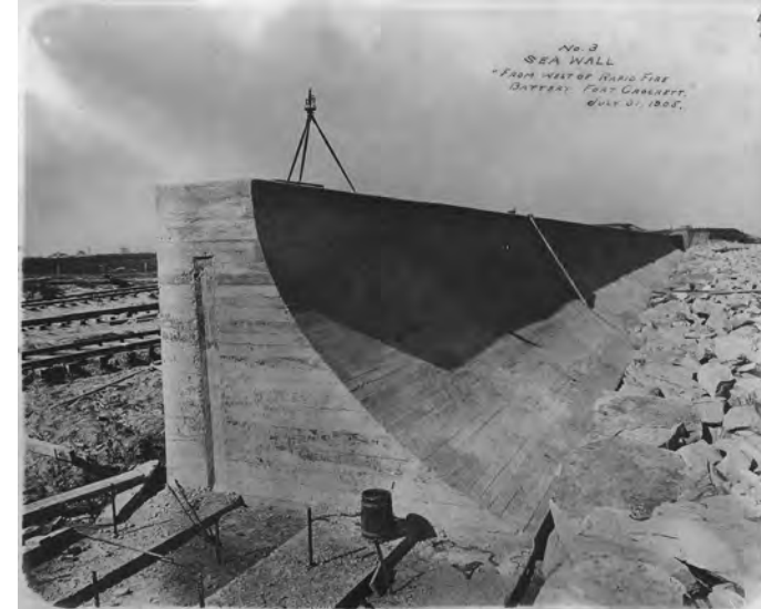
Devastation from the 1900 Hurricane. New seawall under construction in 1906, 15 feet high. (17 above low tide.)
