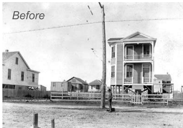
In the before photo, a surviving house has already been raised to the new elevation. A man points to this elevation painted on the utility pole high above his head. In the after photo, the ground level has been filled in below, creating a new, higher ground plane. The man points to the same mark.
