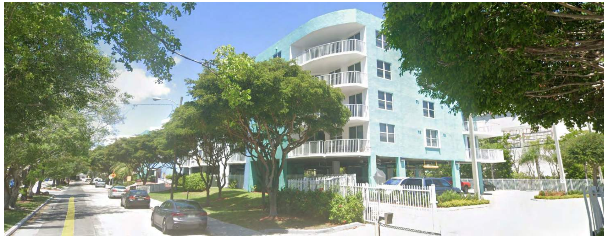
Existing conditions on North Treasure Dr.
