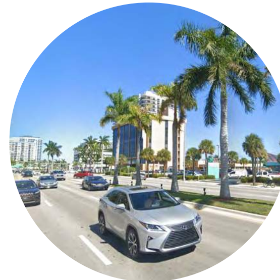
Existing: Kennedy Causeway Inside the R.O.W.
