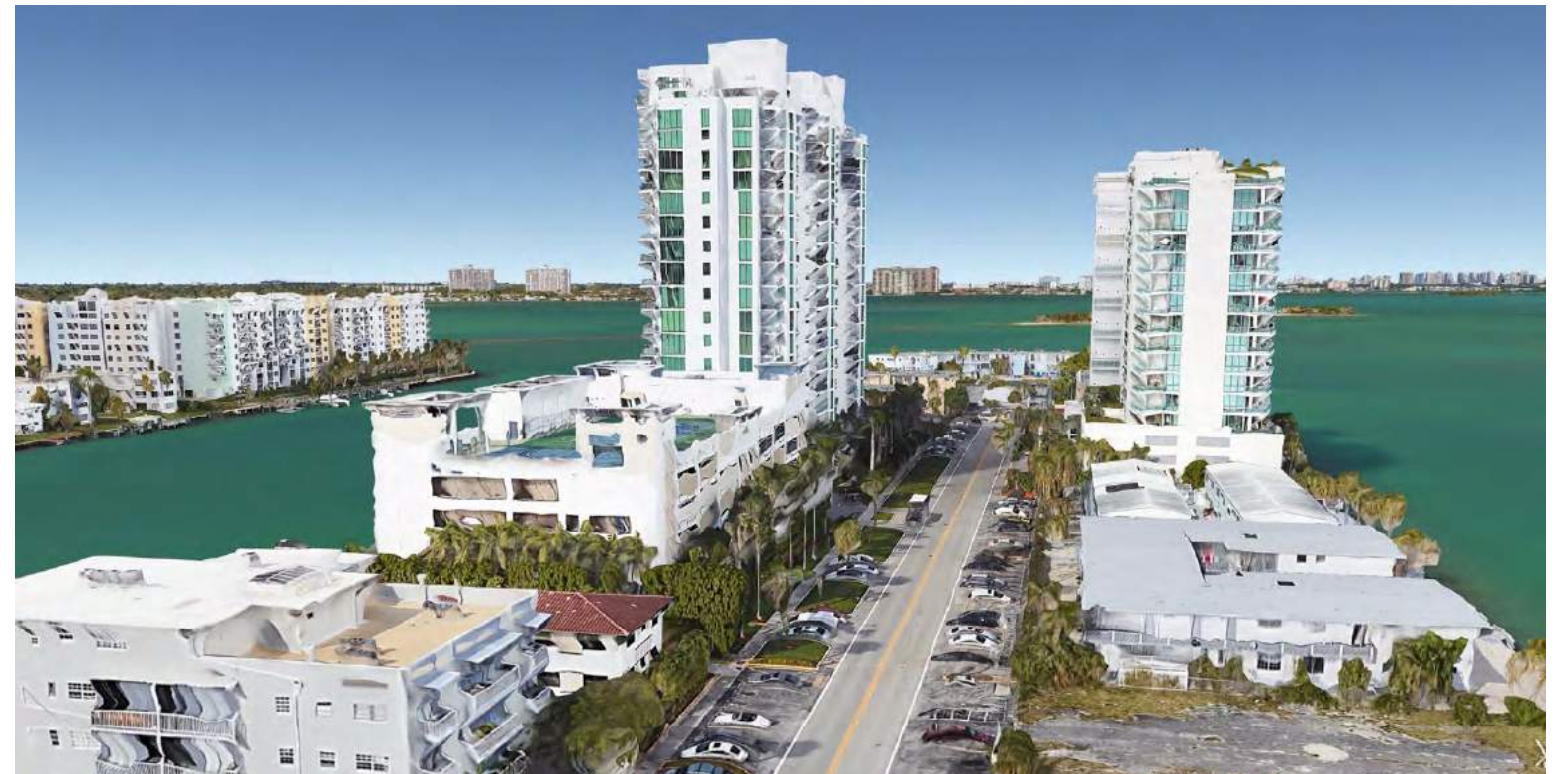
East Drive existing conditions
