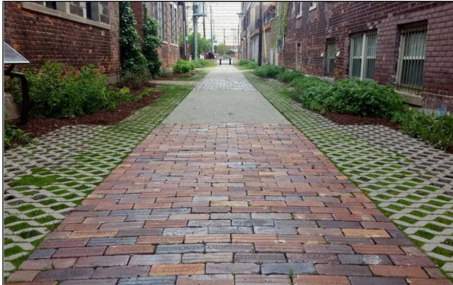
Figure 17 – Green alley in Detroit with pervious pavers
