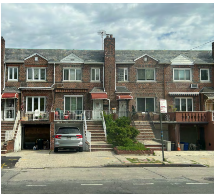
The below-grade garages in the study area are often converted to apartments, which easily flood during significant rain events. (ULI)
