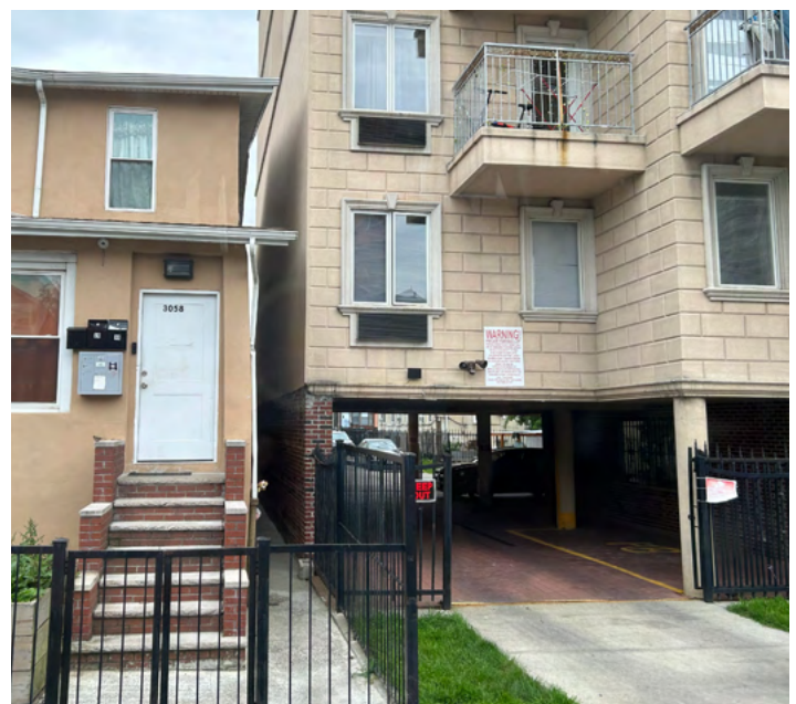
Raising the first level of living space above base flood elevation can ease some of the impacts from flooding. (ULI)
