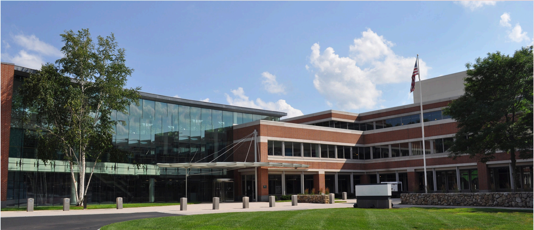
BXP's retrofit of 140 Kendrick Street in Needham, Massachusetts, included VRF heat pumps.
