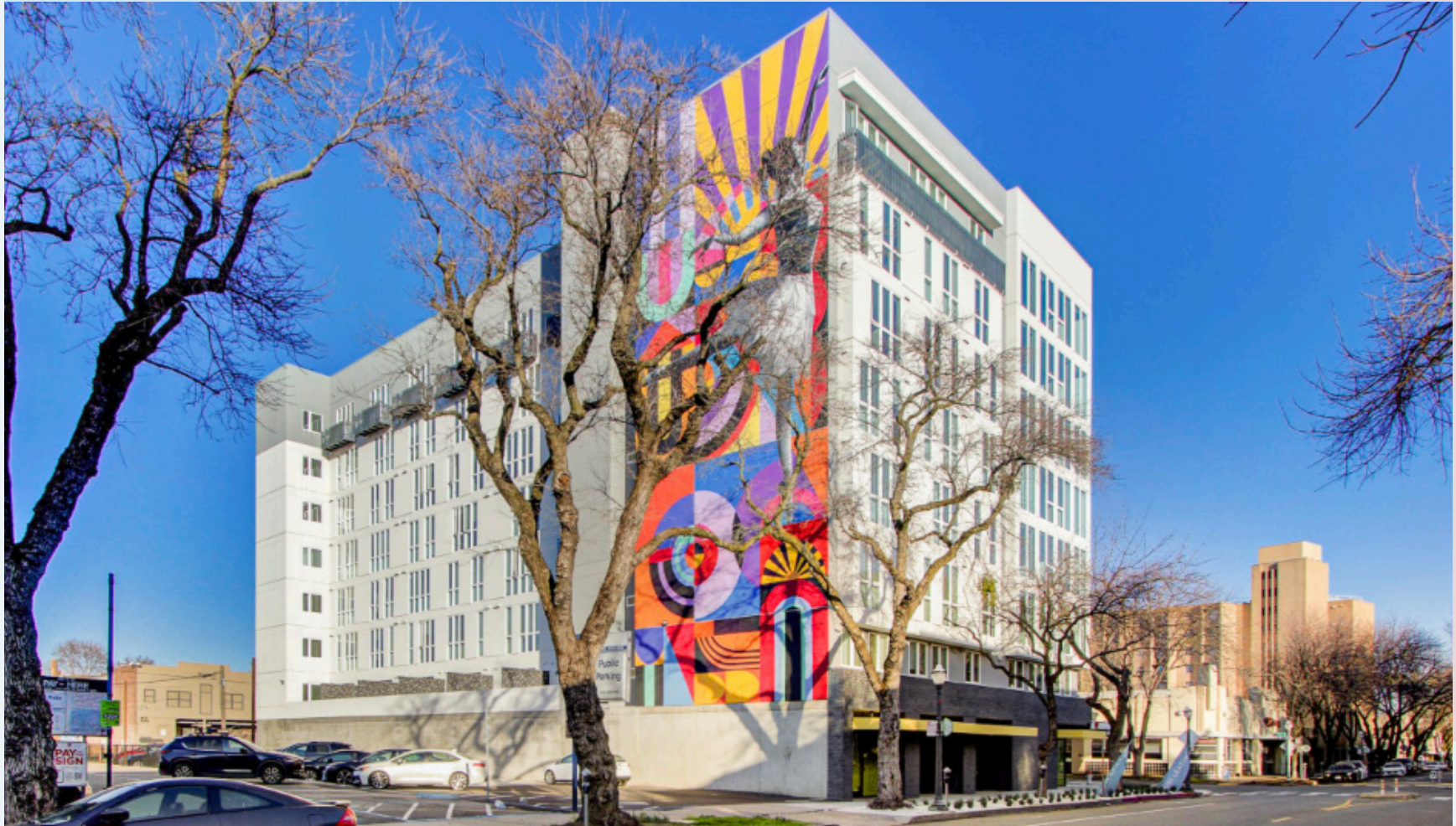
17 Central apartments in Sacramento, California, are conditioned by mini-split heat pumps.
