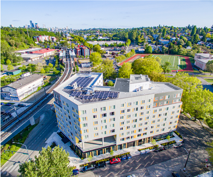
Gardner House in Seattle, Washington, located one block from a light rail station, provides 95 apartments for low-income and formerly homeless families. (Christophe Servieres)
