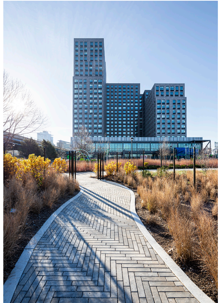
In New York City, Bronx Point is a mixed-use project that took shape on an underused waterfront site in the South Bronx and includes 542 units of permanently affordable housing. (Bronx Point)
