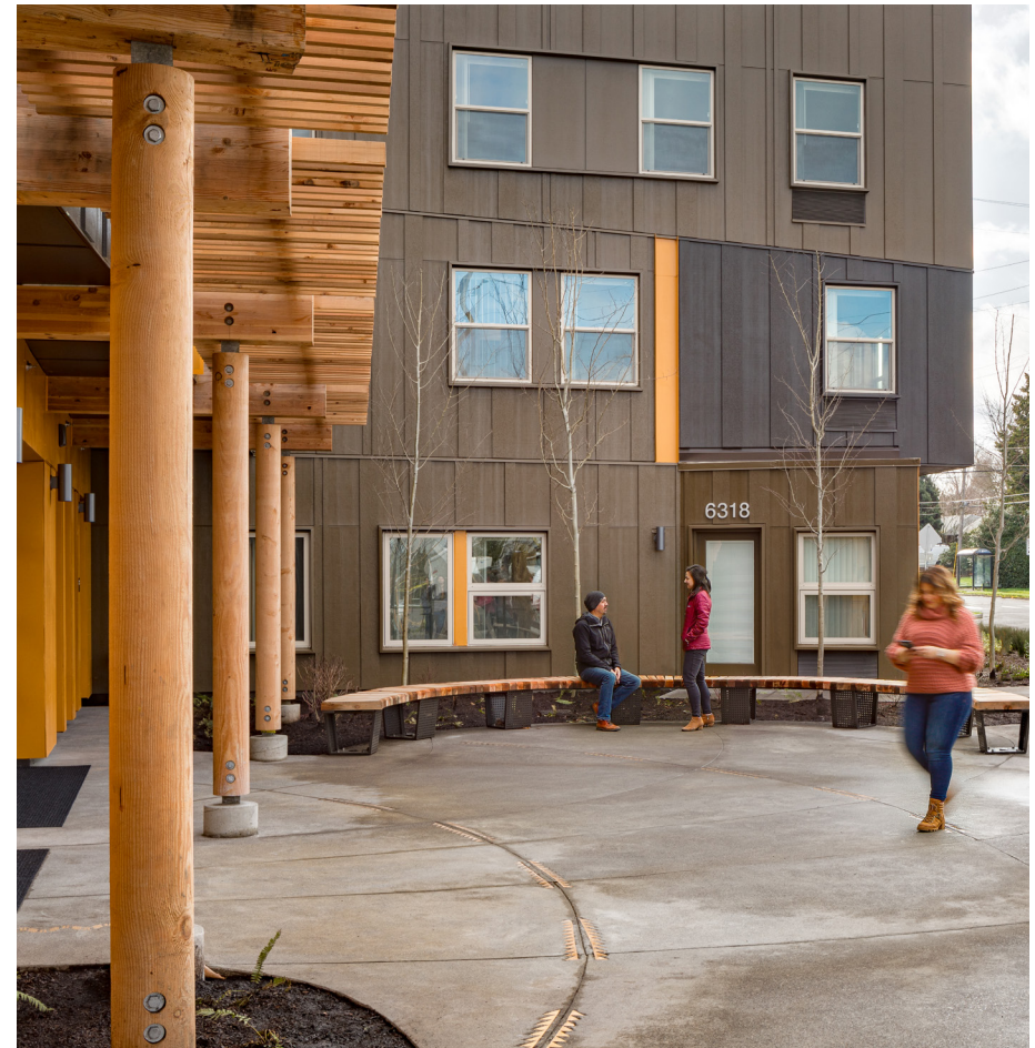
Nesika Illahee offers 59 apartments in Portland, Oregon, with a focus on the needs of the Native community through a partnership with the Native American Youth and Family Center, the Confederated Tribes of Siletz Indians, and the Native American Rehabilitation Association. (Josh Partee Architectural Photographer)
