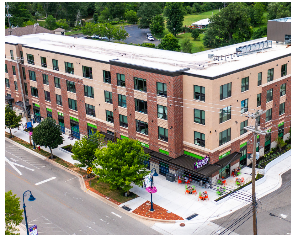
Broadway Lofts created 48 affordable apartments and a mixed-use development on a former brownfield site in Mount Pleasant, Michigan. (Michigan Community Capital)
