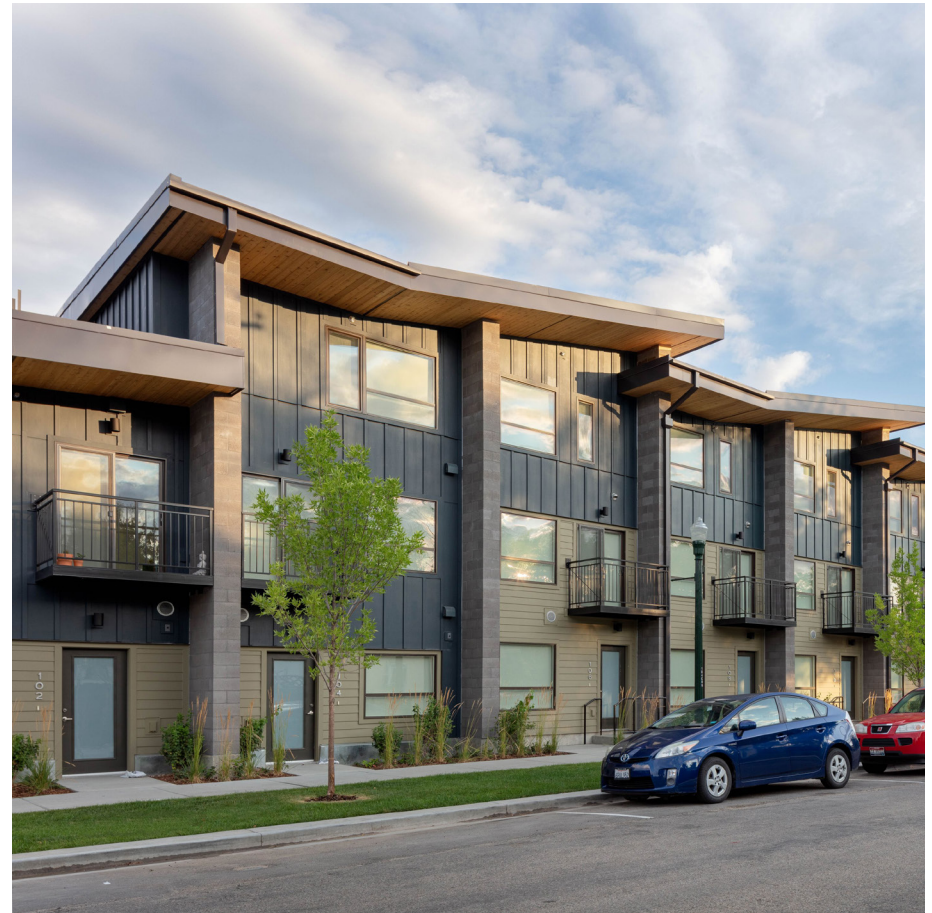
Ash+River Townhomes in Boise, Idaho, is 34 units of workforce/moderate-income housing near the city's downtown. (Nate Stallings for deChase Miksis)
