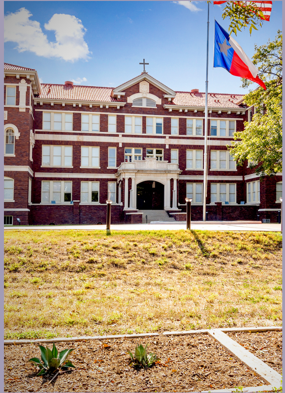
The adaptive use of the former St. John's Seminary in San Antonio, Texas, created 228 apartment homes for a range of income levels. (Paige Shinn Photography)
