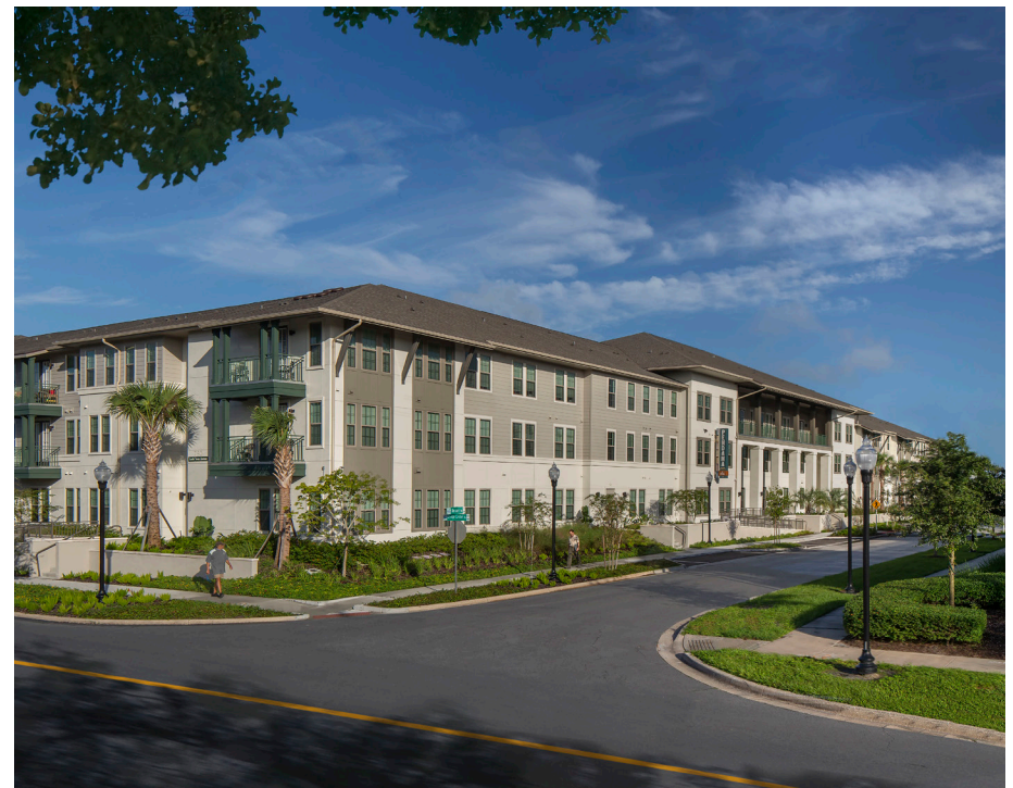
Pendana at West Lakes is the rehabilitation of hundreds of vacant and dilapidated apartments into a mixed-use, mixed-income community with 320 apartments near downtown Orlando, Florida. (Rion Rizxo/Creative Sources)
