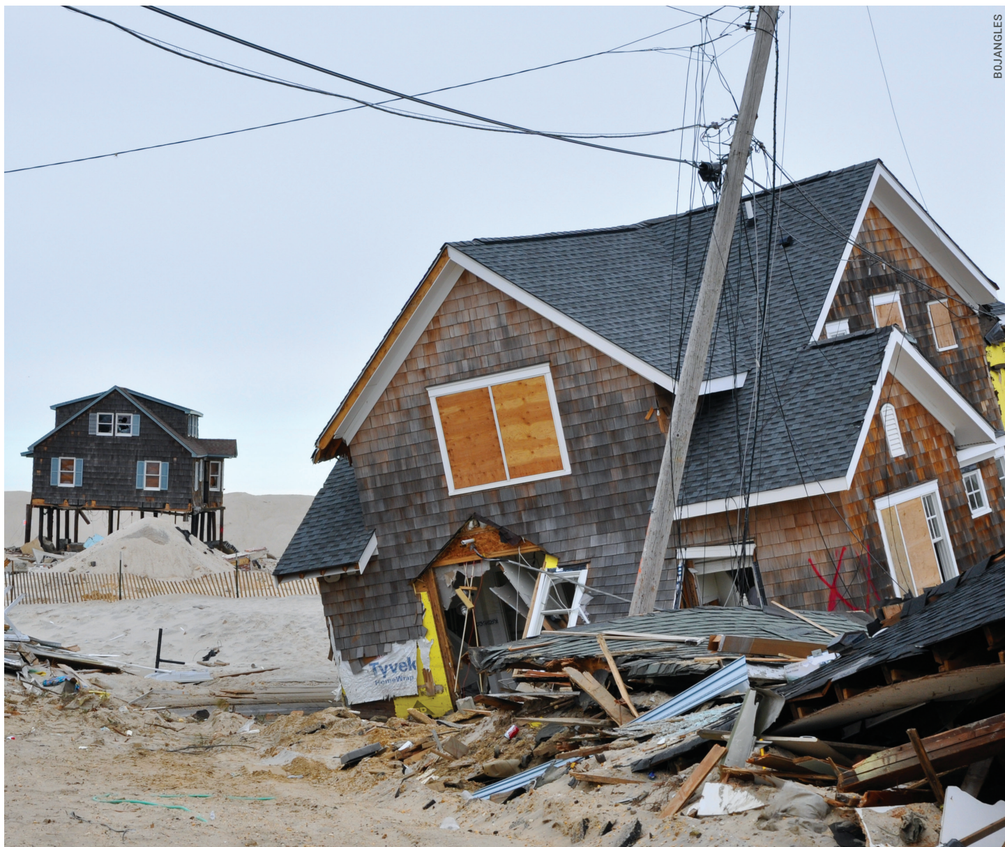
Damaged properties in Ortley Beach, New Jersey, following Hurricane Sandy.
