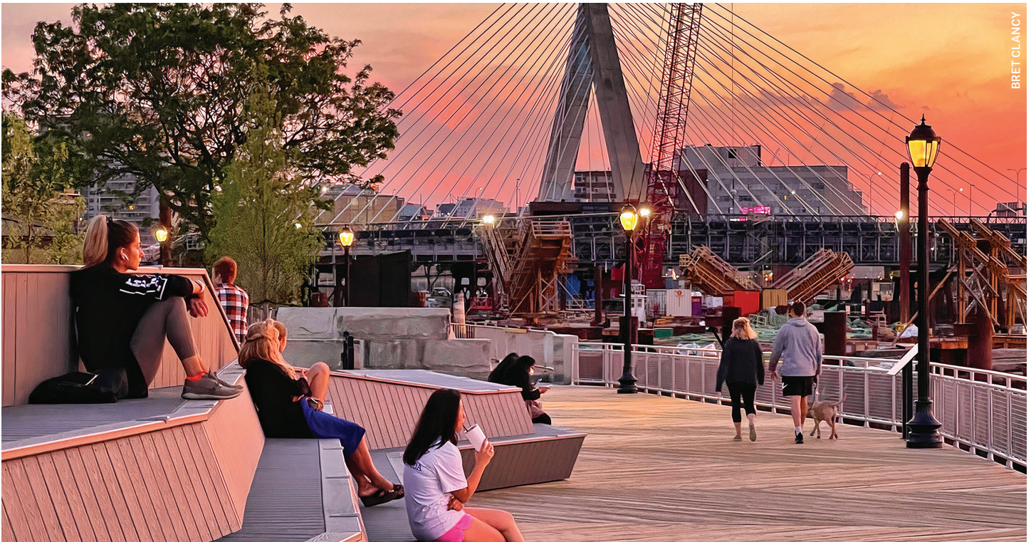
The secondary sea wall at Langone Park and Puopolo Playground in Boston, Massachusetts, offers overlooks and seating with expansive harbor views, while breaks in the wall allow people to get down to the harbor and some water to enter and leave the site. The new sea wall's foundation is designed to hold additional weight so that it can be built upon if flood projections change in the future.
