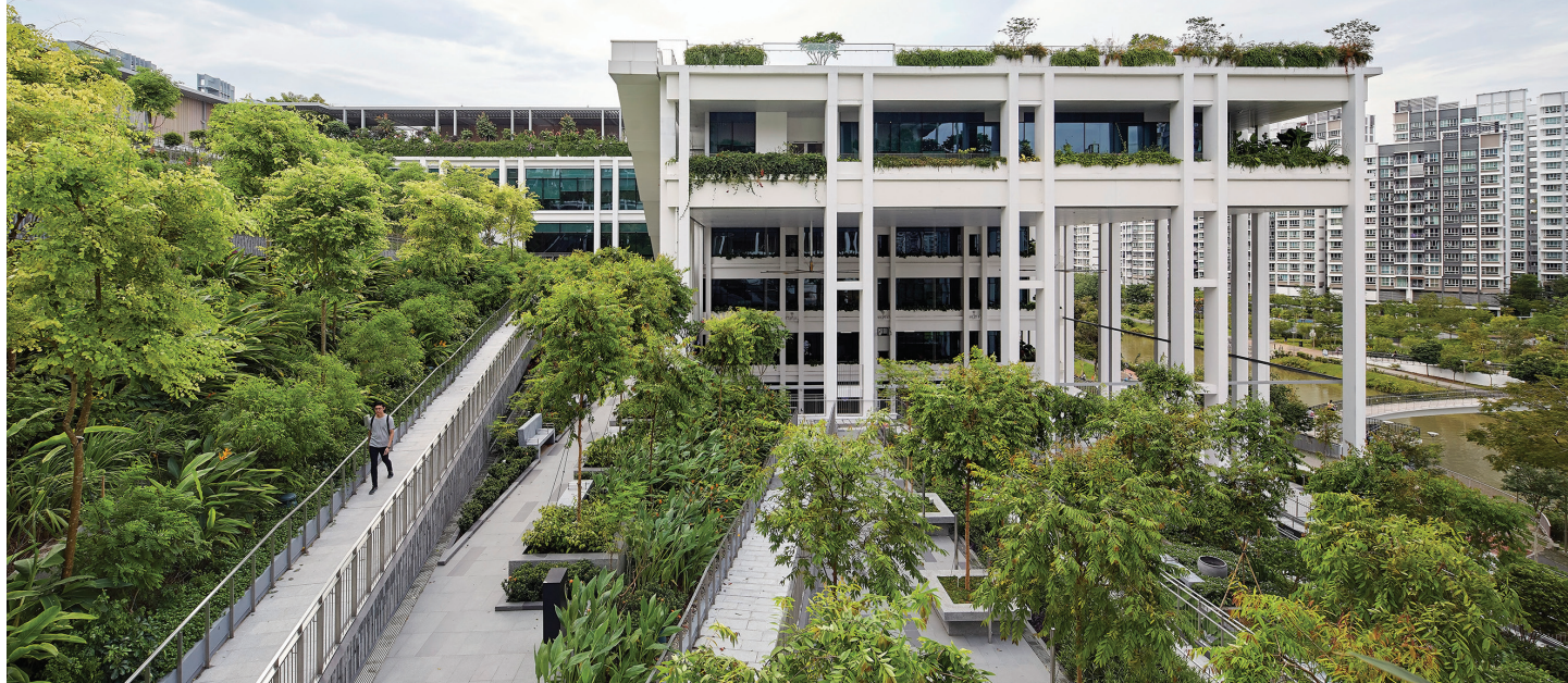
Oasis Terraces is richly planted with terrace greenery maintained by neighborhood residents. The plants help to absorb stormwater and cool the building from Singapore's rising heat.
