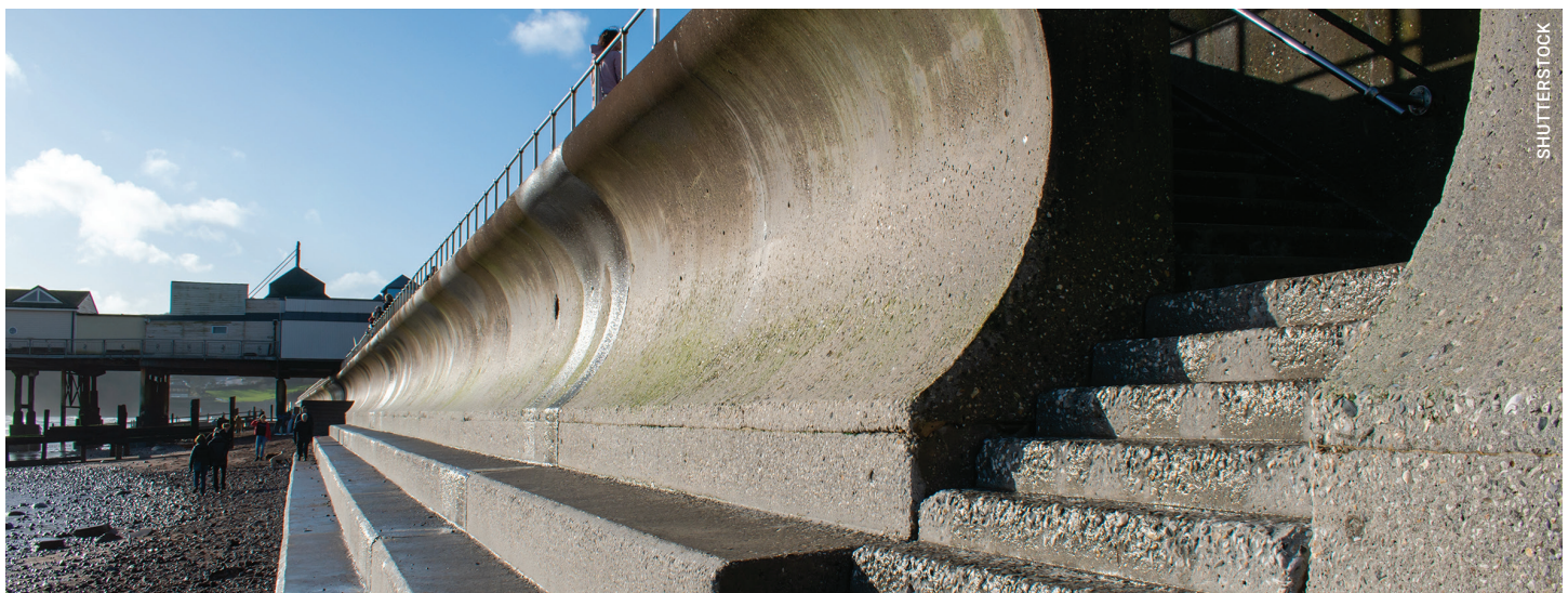
Curved sea walls are more effective at dissipating wave energy than vertical walls, which means they may take less damage.
