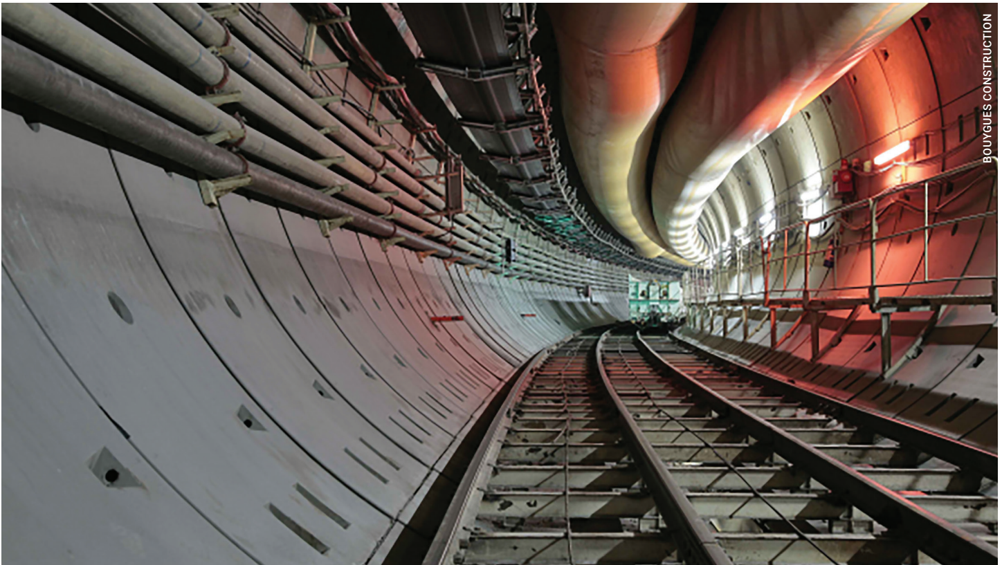
Hong Kong's west drainage tunnel collects stormwater with 32 wells and linking tunnels that expel the water into the sea.
