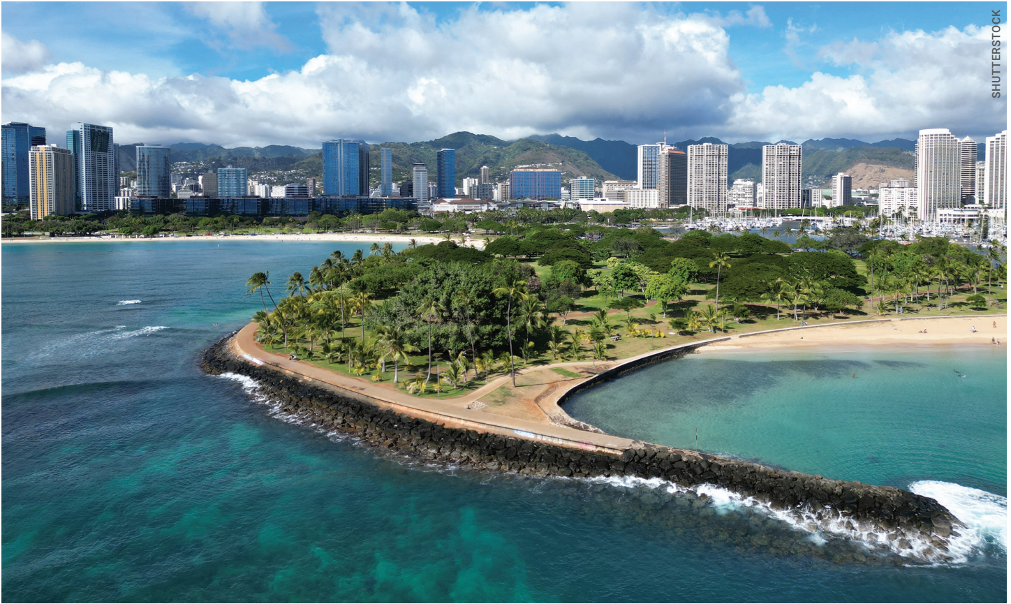
Breakwater at Magic Island, O'ahu, Hawaii.
