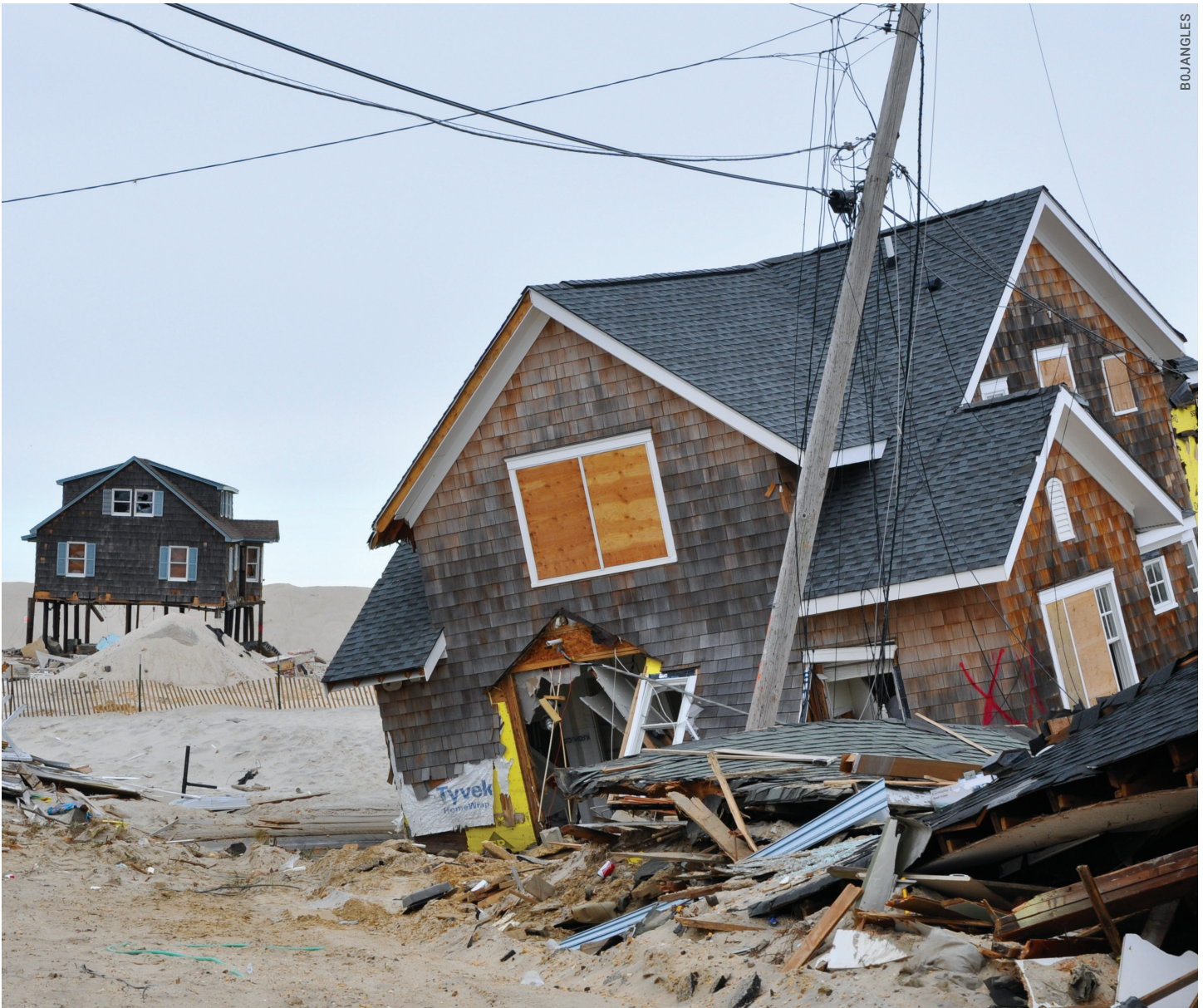
Damaged properties in Ortley Beach, New Jersey, following Hurricane Sandy.
