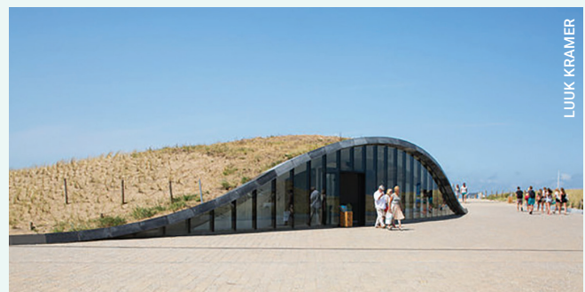
An underground parking garage , embedded seamlessly amidst the dunes of the seaside resort town Katwijk aan Zee, protects the coastline while providing access to the shore.
