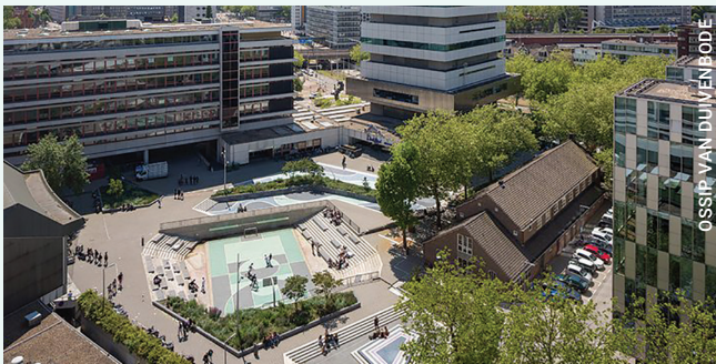
The Bentheplein, or Water Square , a public park in Rotterdam by De Urbanisten, uses sunken sport courts to double as recreational space and stormwater storage.
