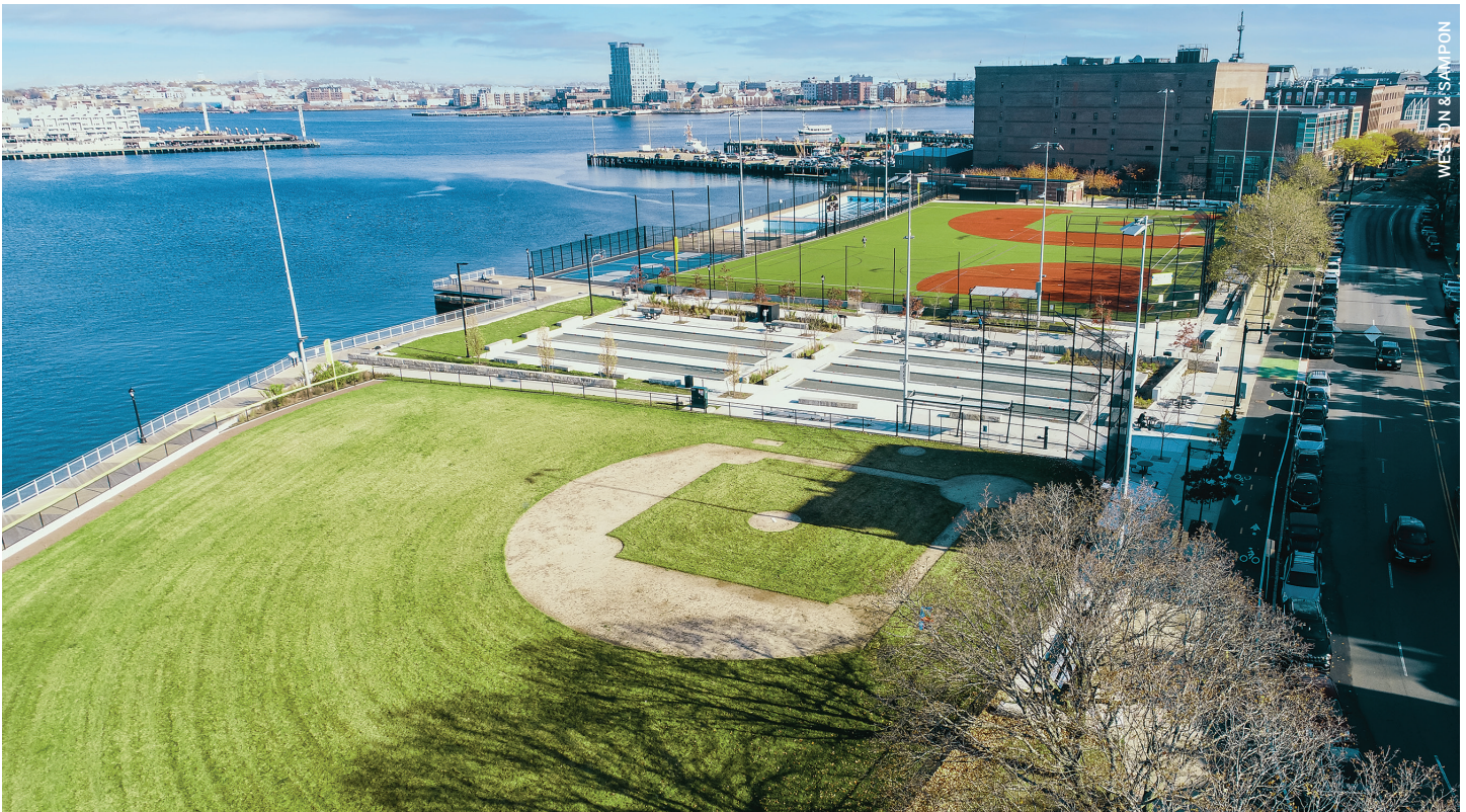
Langone Park and Puopolo Playground in Boston, Massachusetts, protects the surrounding community from sea level rise and flooding while preserving access to the waterfront. In an adaptive approach, a second sea wall was constructed behind an existing sea wall to add protection to the site. The approach greatly reduced permitting and construction complexities, and the wall works effectively as a wave action barrier.
