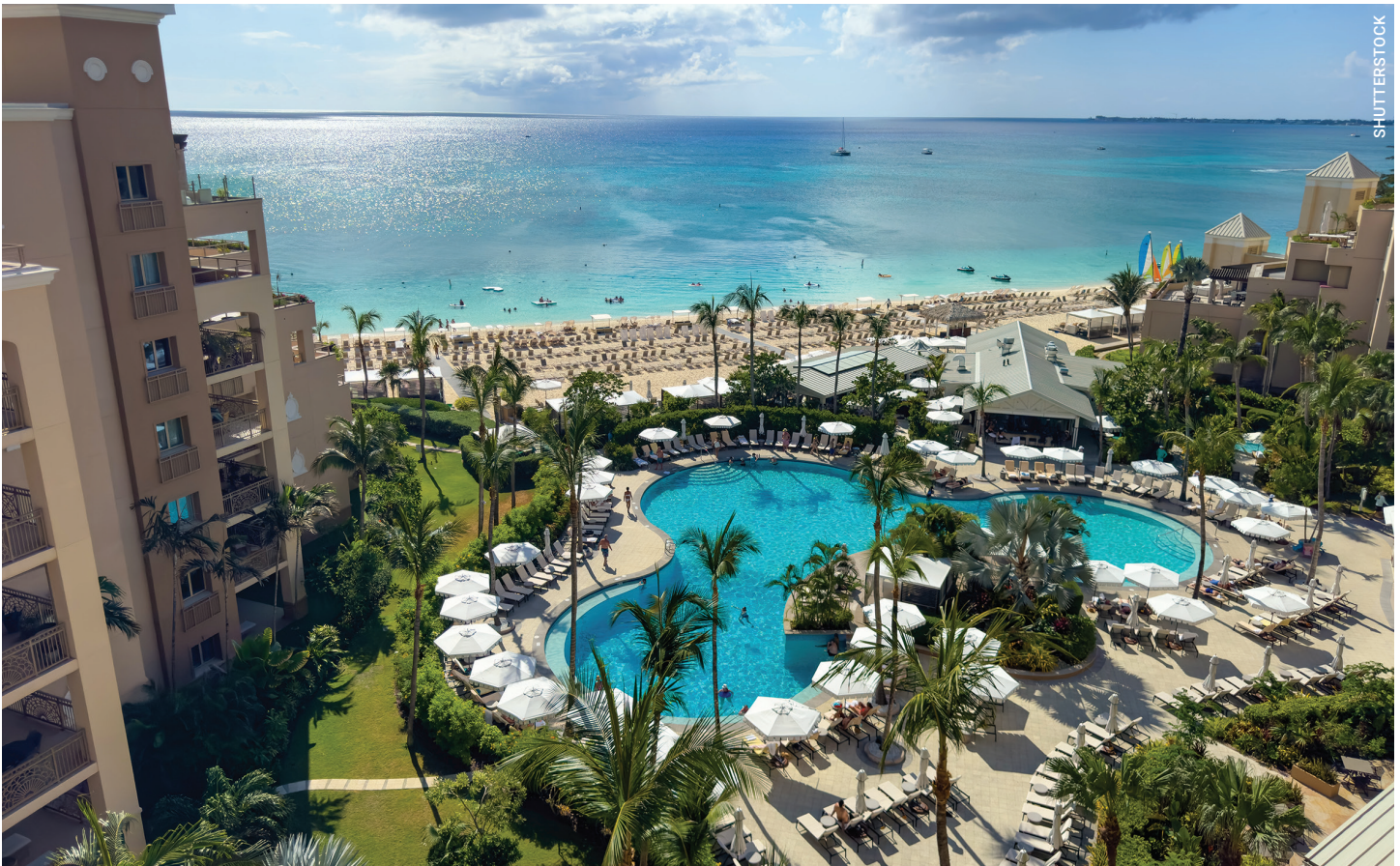
The Ritz-Carlton in Grand Cayman. After damage from Hurricane Ivan in 2004, new owners Five Mile Capital Partners installed multiple building and landscape resilience measures for coastal storms, including mangrove restoration. They note these features have enhanced property value, reduced annual utility costs by $300,000, and provide attractive and unique amenities, all while supporting their relationship with local government.
