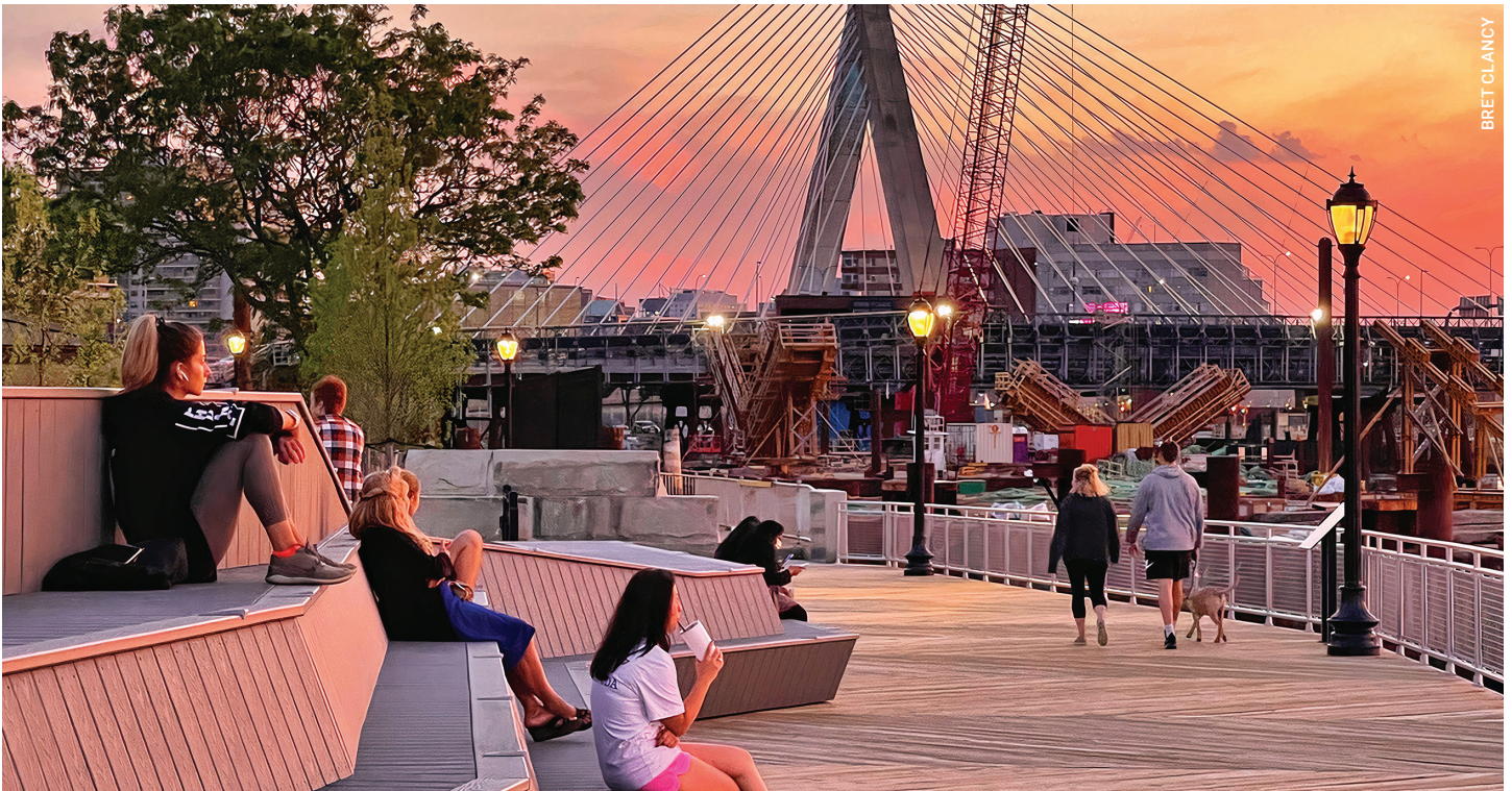
The secondary sea wall at Langone Park and Puopolo Playground in Boston, Massachusetts, offers overlooks and seating with expansive harbor views, while breaks in the wall allow people to get down to the harbor and some water to enter and leave the site. The new sea wall's foundation is designed to hold additional weight so that it can be built upon if flood projections change in the future.
