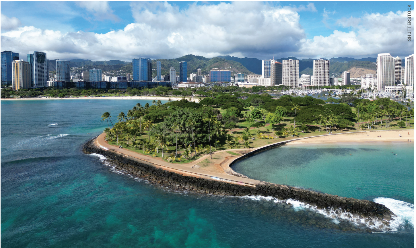
Breakwater at Magic Island, O'ahu, Hawaii.
