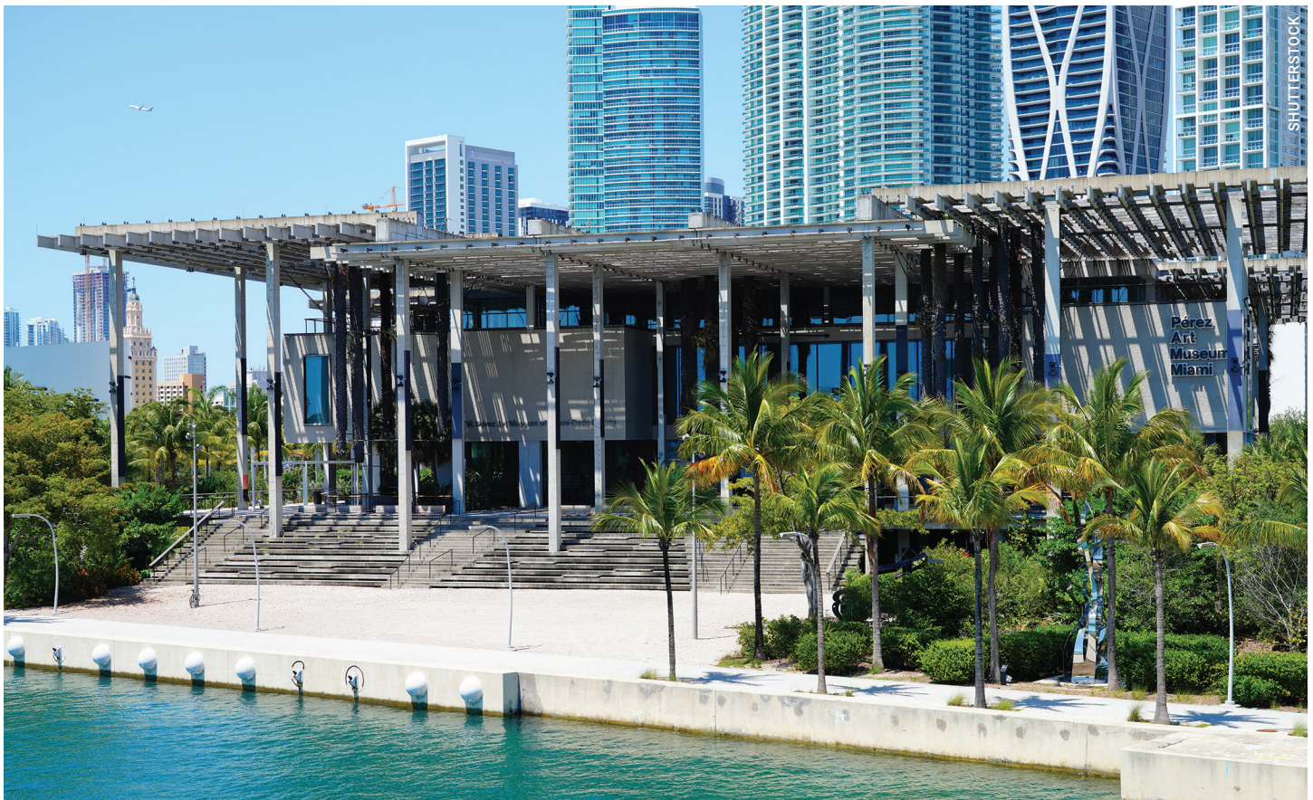
The Pérez Art Museum in Miami, Florida, is raised to allow a flood surge from Biscayne Bay to flow underneath, providing viewing terraces for museumgoers.
