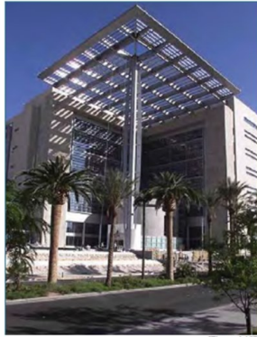
[Figure 4.127] Federal Courthouse in Las Vegas, Nevada.
