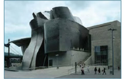
[Figure 4.128] Guggenheim Museum in Bilbao, Spain.
