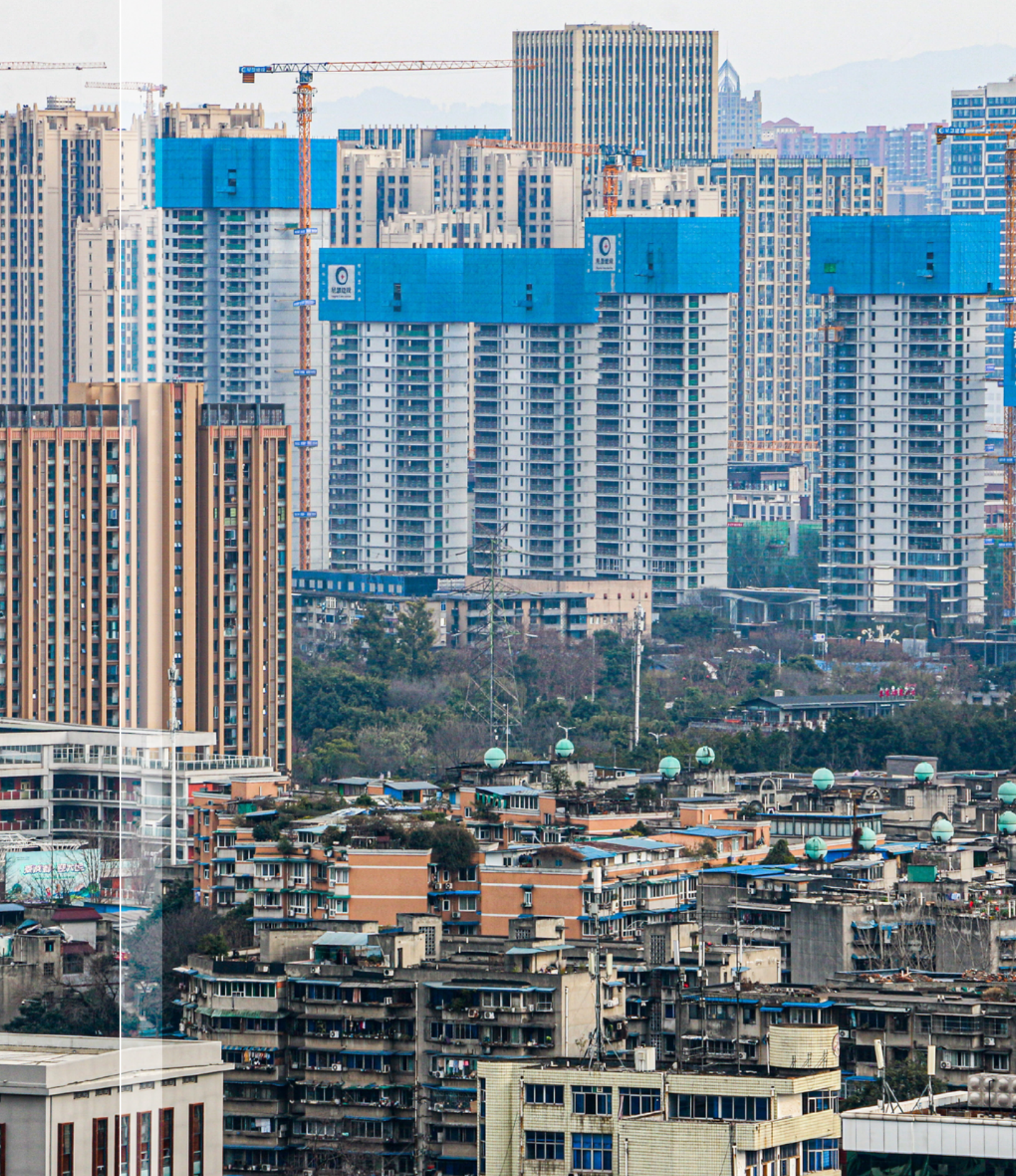
High-rise residential buildings being built in Chengdu, China. Credit: Shutterstock
