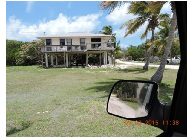
Resident Manager Building
