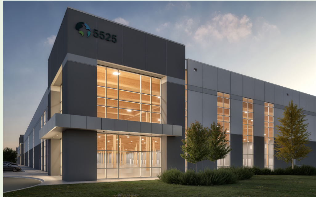
Prologis Evergreen combines mass timber and prefabricated concrete panels to reduce the embodied carbon of the structure.
