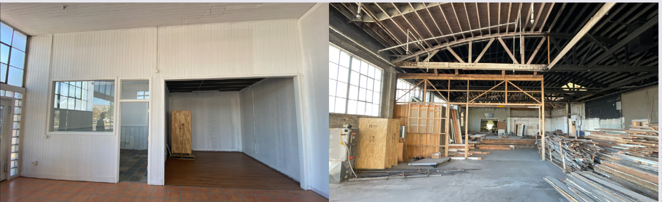
Watershed Row and its sister project, Wood River Mercantile, have undergone careful deconstruction, instead of demolition, to salvage materials. These images depict Watershed Row before and after deconstruction.
