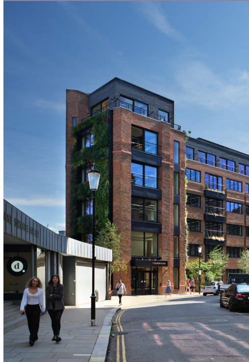
The development of Holbein Gardens followed circular economy principles by preserving the original structure, reusing materials, and diverting 99 percent of site waste from the landfill.
