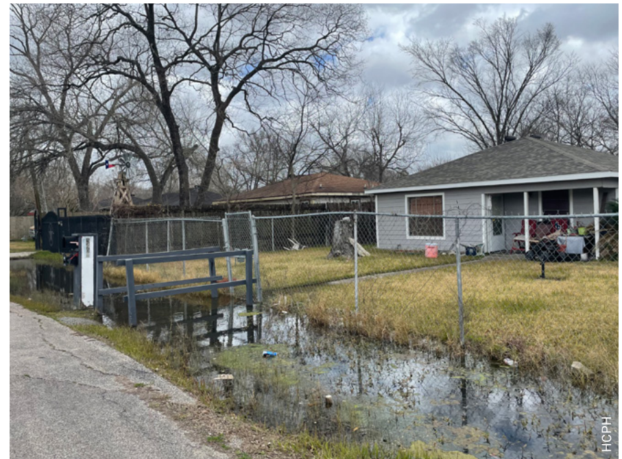
Figure 8. A flooded drainage ditch filled with trash in Settegast. The flooding is preventing access to this home.
