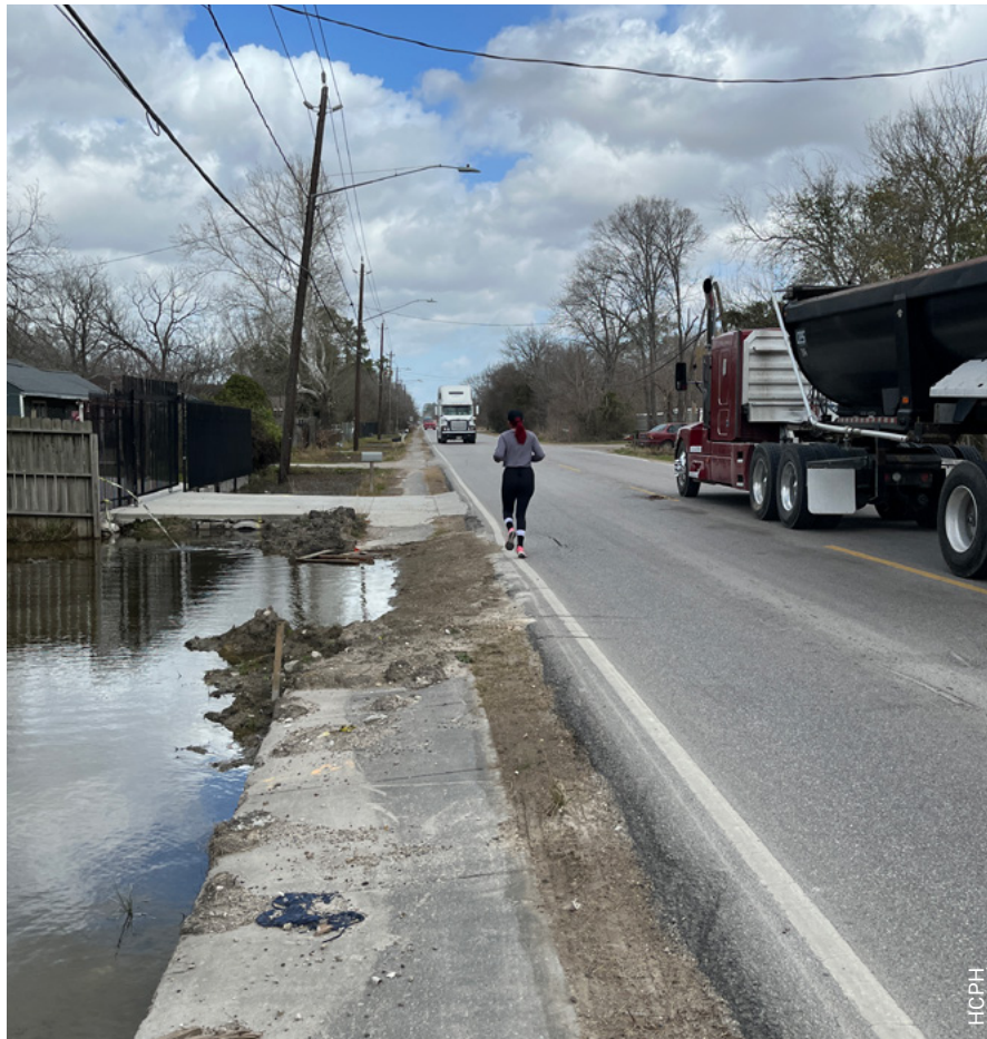
Figure 7. A damaged sidewalk forces a woman to run on a narrow road next to 18-wheeler trucks.
