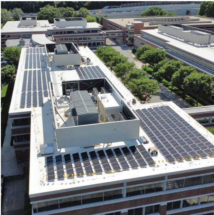
Solar panels on Building A. (Courtesy of BXP)
