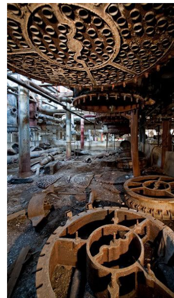
An interior view of the Great Western Sugar Mill. Photo courtesy Scott Haefner.
