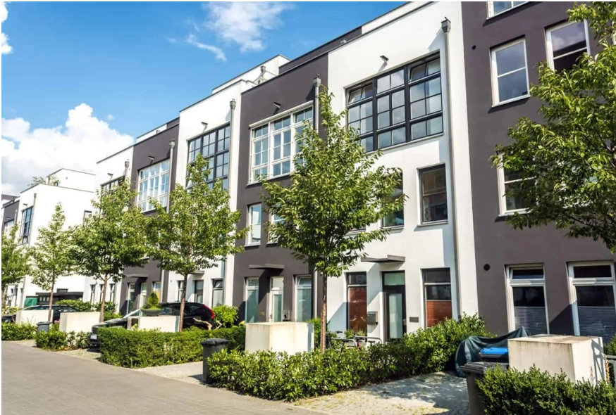
Modern apartment buildings in Berlin, Germany. Photo by querbeet.
