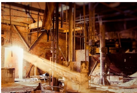
An interior view of the Great Western Sugar Mill. Photo courtesy SUBSTREET.
