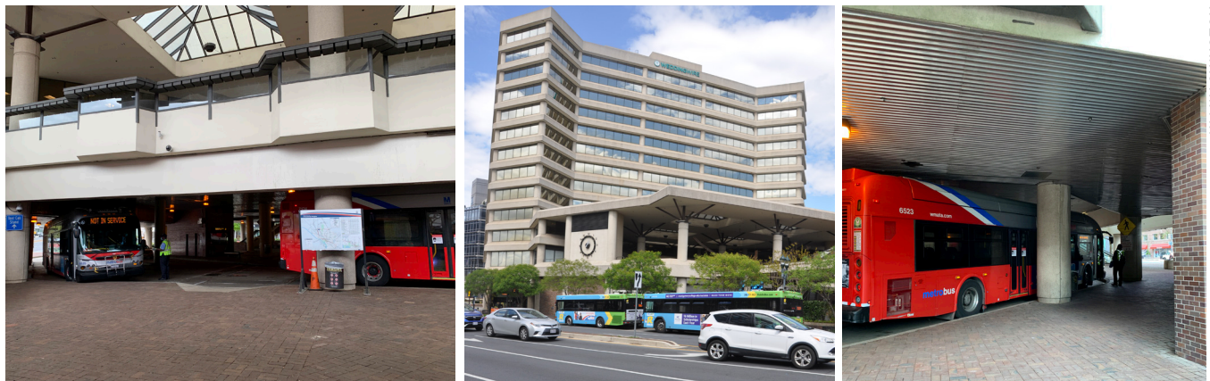
Existing bus loop at the intersection of Wisconsin Avenue and Western Avenue.
