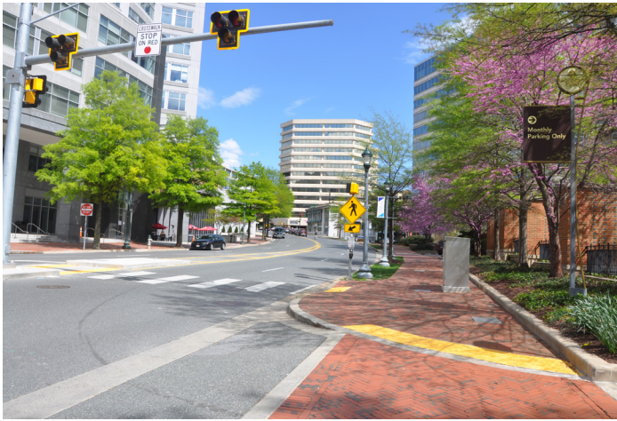
View along Willard Avenue, looking towards Wisconsin Avenue.
