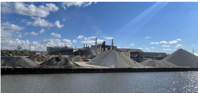
Bulkheads along more industrialized property on the Cuyahoga River. Industrial spaces tended to have bulkheads in much better conditions compared to private and public property due to operational necessity for property owners.
