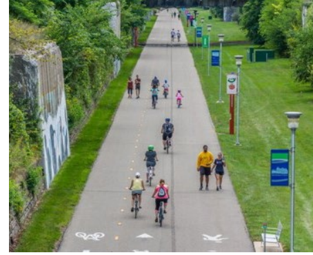
The Dequindre Cut in Detroit provides an example of separated lanes on a trail. Photo courtesy DetroitRiverfront.org.
