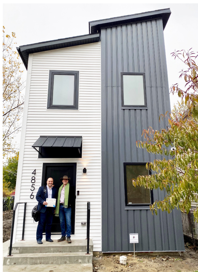
Modular Home in Chicago's Back of the Yards Neighborhood.
