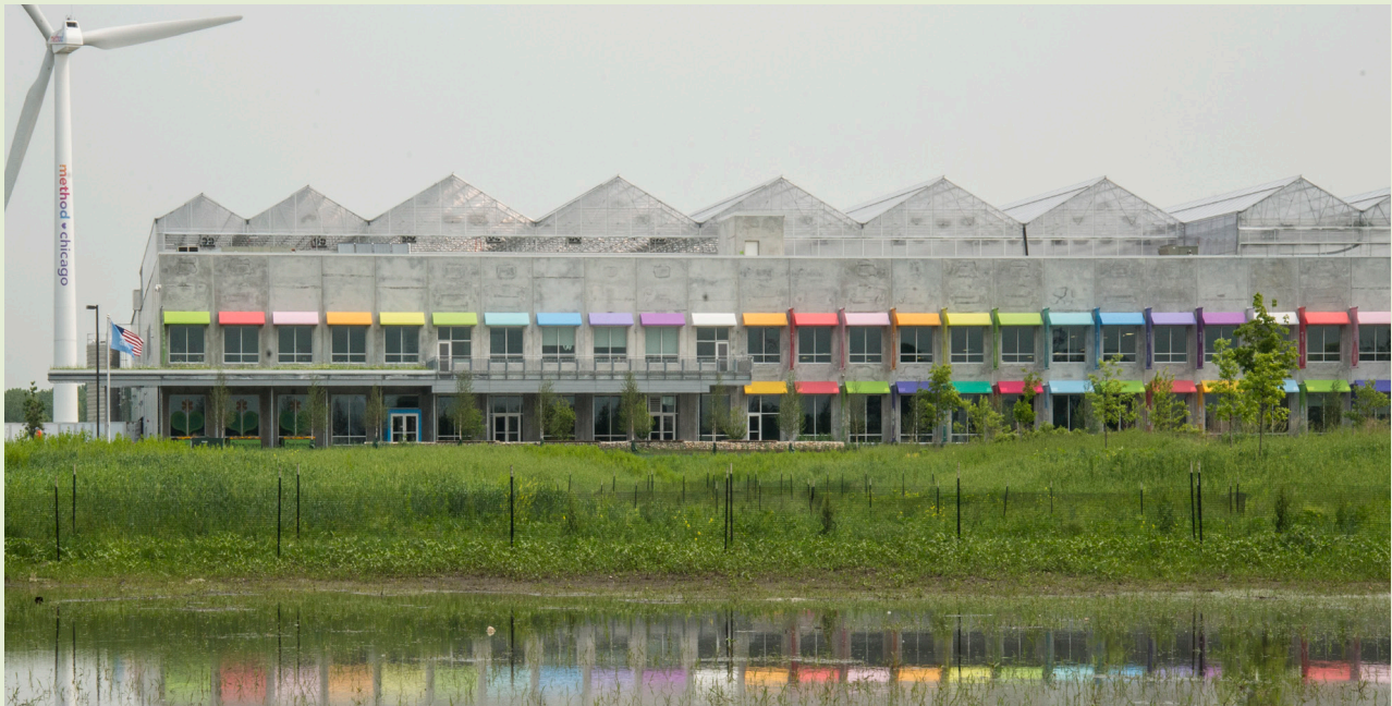
Method Plant and Gotham Greens, Pullman Park.
