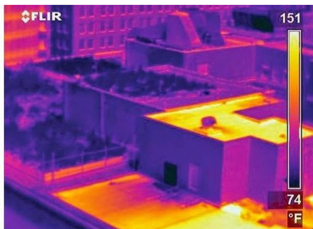
The Chicago City Hall green roof measures almost 80°F cooler than the other sections of the roof that have not been improved with the green infrastructure.
