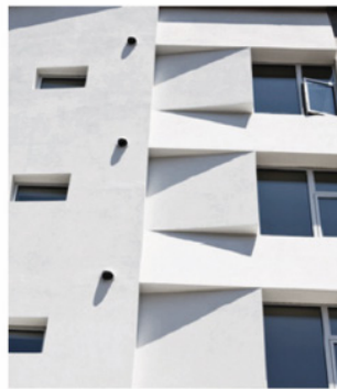
EIFs Insulation wedges with ERV ducts
