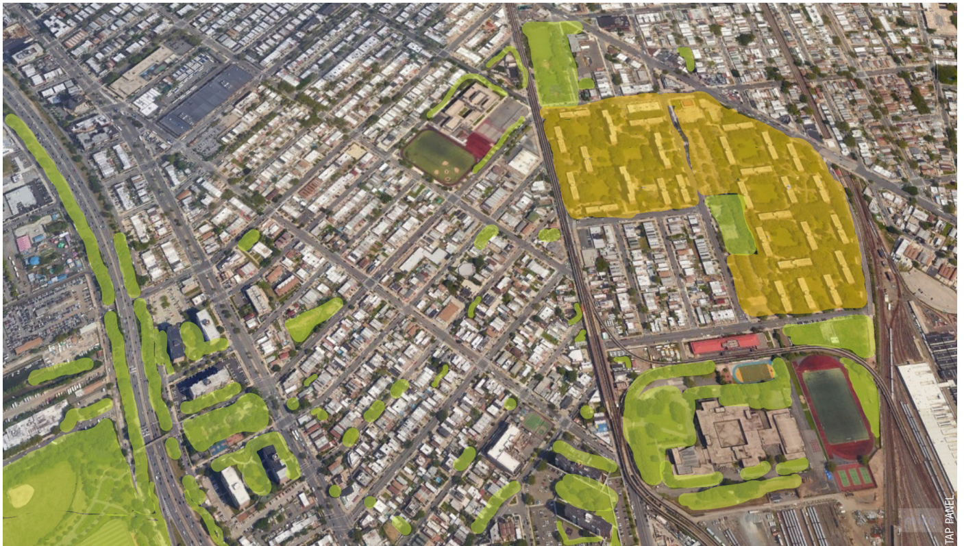
Caption: Marlboro Houses (in yellow) is surrounded by significant green infrastructure (in green) that can create a linked corridor network, providing even greater ecosystem services like cooling and stormwater management. Source: Google Maps and TAP Panel.
