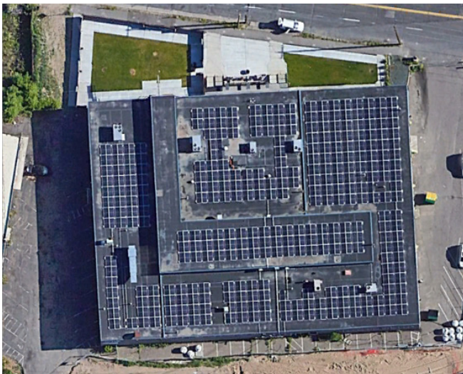
View of the Solar Installation on the roof of the Glass House Building in the Root District.
