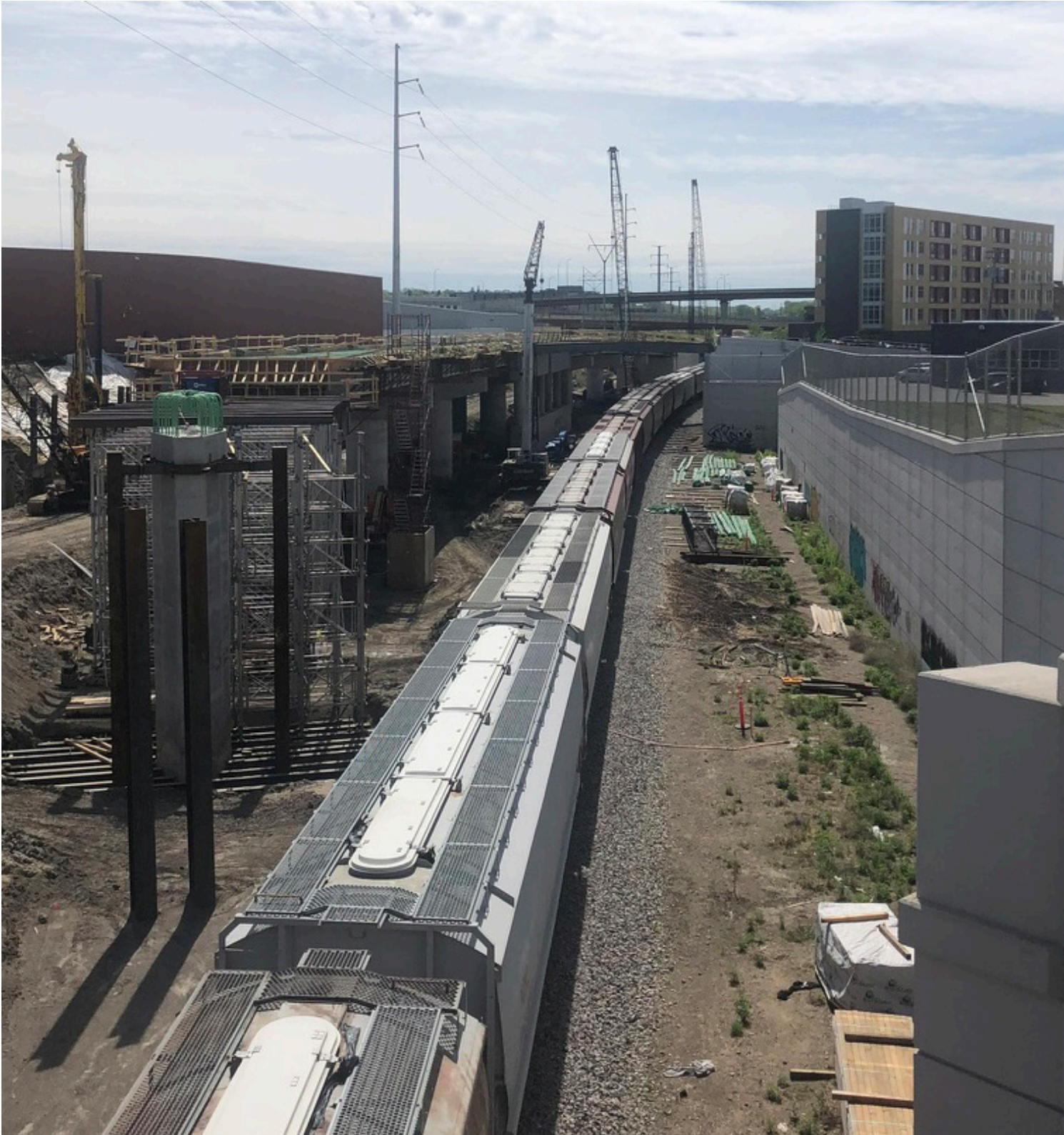
View of Green Line LRT construction through the Root District.
