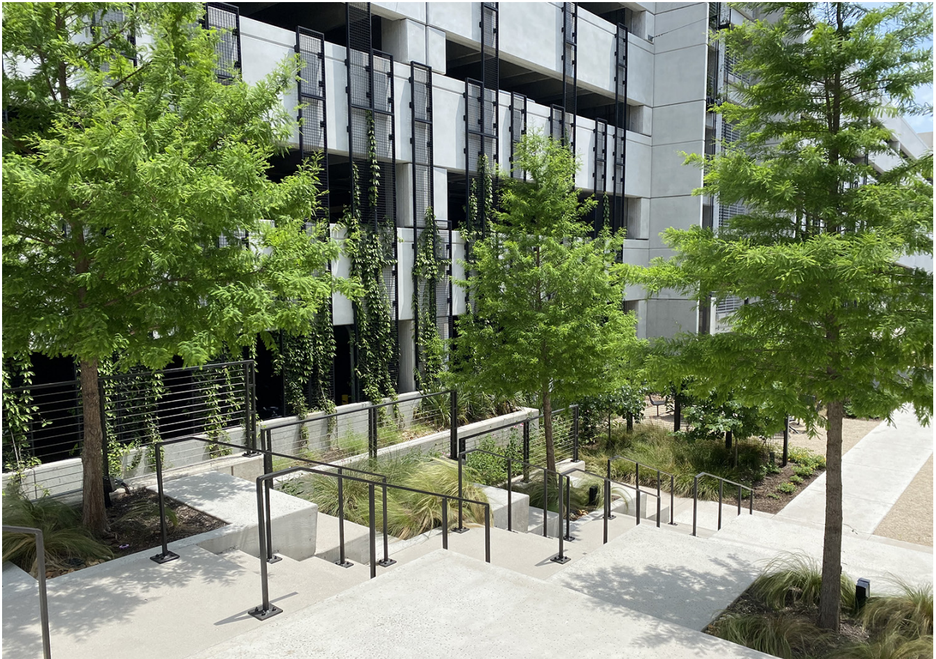
The City of Austin is leading by example by moving the operations of the building and permitting departments to a building and campus that feature a variety of green building practices and products.
