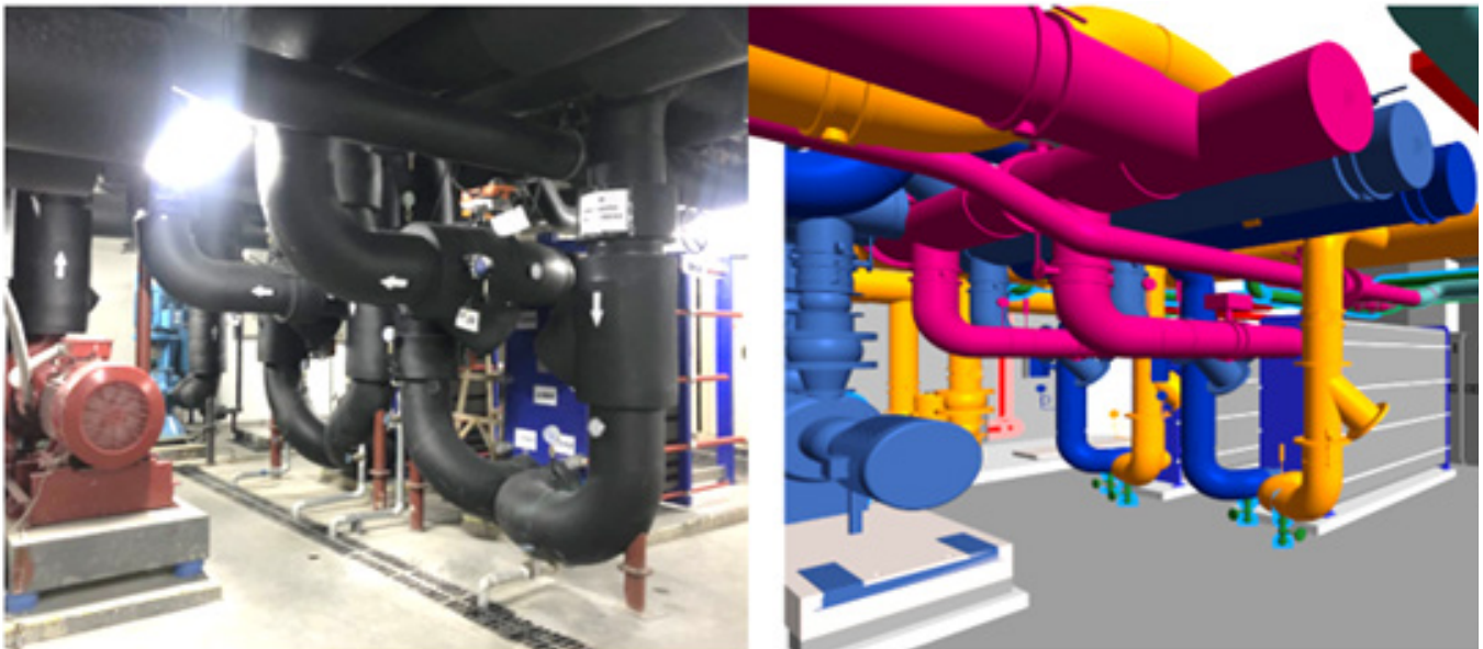
Figure 13 – BIM Model of Plant Piping Network
