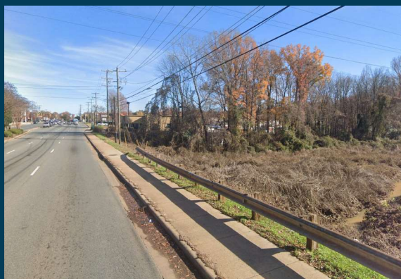
Albemarle Road's existing sidewalk conditions.
