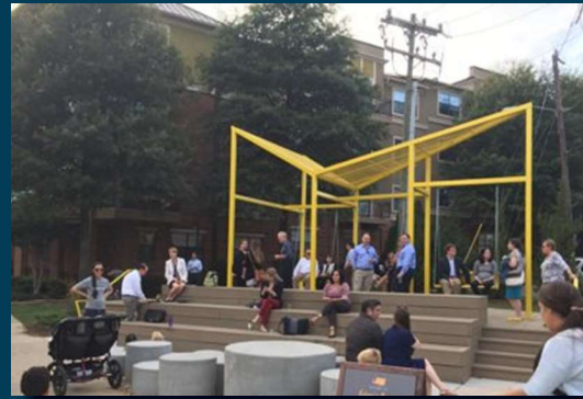
After picture of Edna's Porch along the Lynx Blue Line Light Rail.
