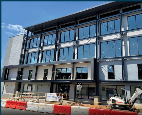
Commercial office building along The Plaza Road with modern upfits such as low-E glass windows.
