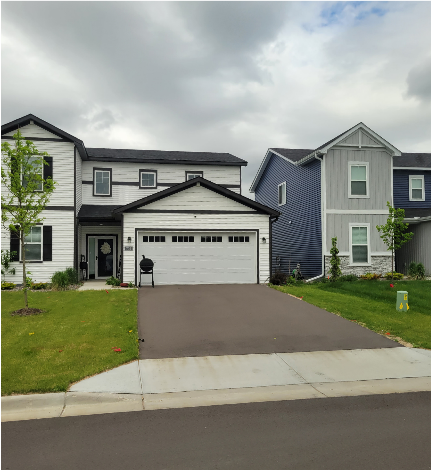
Recent housing development, Brooklyn Center, Minnesota. (Urban Land Institute)
