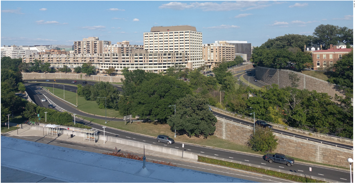
I-66 Infrastructure as seen from the Kennedy Center Roof Terrace.
