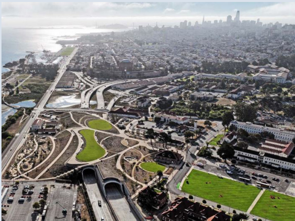
The Presidio Tunnel Tops.
