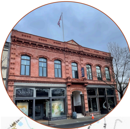
Site tour image of one of St. Helena's signature historic buildings on Main Street.
