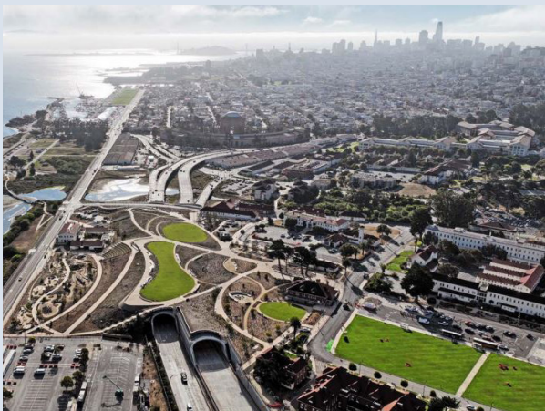
The Presidio Tunnel Tops.
