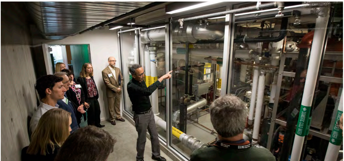
The Bullitt Center in Seattle is a six-story, 44,700 square foot office building designed to meet the stringent requirements of the Living Building Challenge (LBC) . Visitors to the center are learning about the building’s geothermal heating and cooling system that operates on electricity generated by solar panels on the building rooftop. More information on Bullitt Center’s green features is included in the ULI Case Study .
