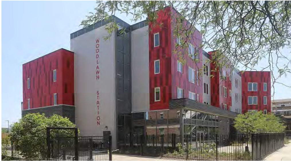
Located at the entrance to the CTA's Green Line station at 63rd Street and Cottage Grove Avenue, Woodlawn Station by POAH Chicago features 55 mixed-income units. The four-story building has many sustainable features including a solar thermal system, enhanced insulation, and a tight building envelope.
