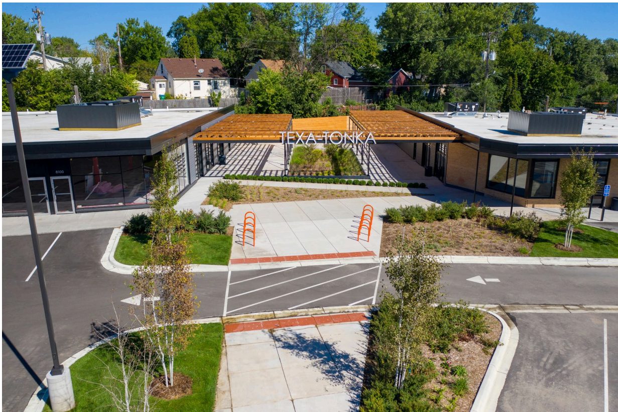
The idea for a restaurant with plaza was inspired by the Texa-Tonka project in St. Louis Park, which offers a compelling atmosphere for gathering. Photos courtesy of Paster Properties.
