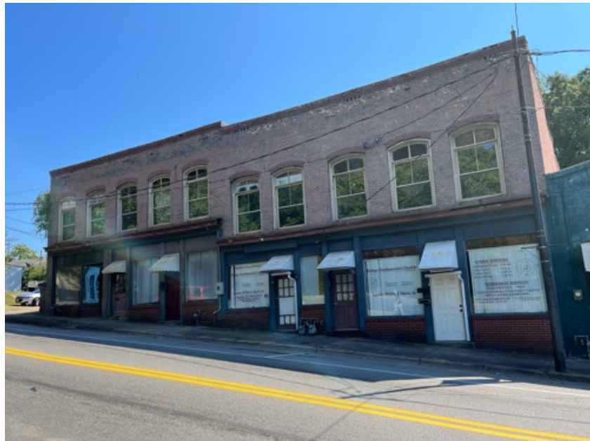
Image 3: North Main Facades. Existing Storefront
