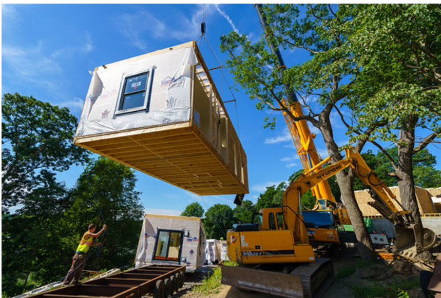
Modular construction, a process in which significant portions of a building are constructed offsite in a controlled environment and then assembled on site, can reduce building costs and construction timelines.
