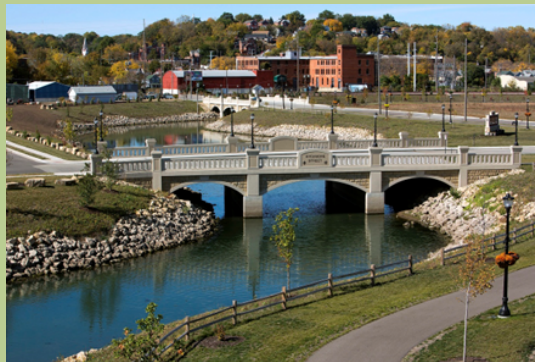
The City of Dubuque, Iowa's Bee Branch Creek Restoration involved replacing almost one mile of storm sewers with a creek and floodplain similar to one that existed a century ago. This allows stormwater from flash floods to move through the area without flooding adjacent properties. https://www.cityofdubuque.org/804/Bee-Branch-Creek-Restoration
