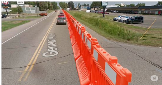
Example of temporary barriers to protect pedestrians.
