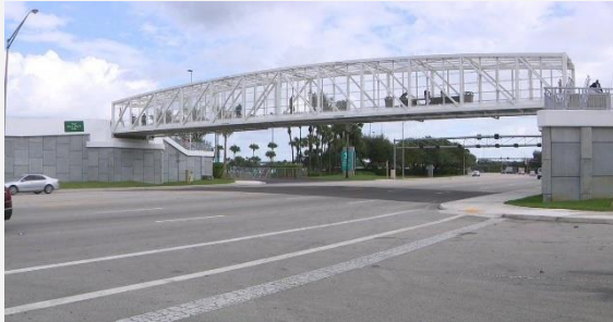
Pedestrian Bridge - Hard Rock Stadium, Miami, FL
