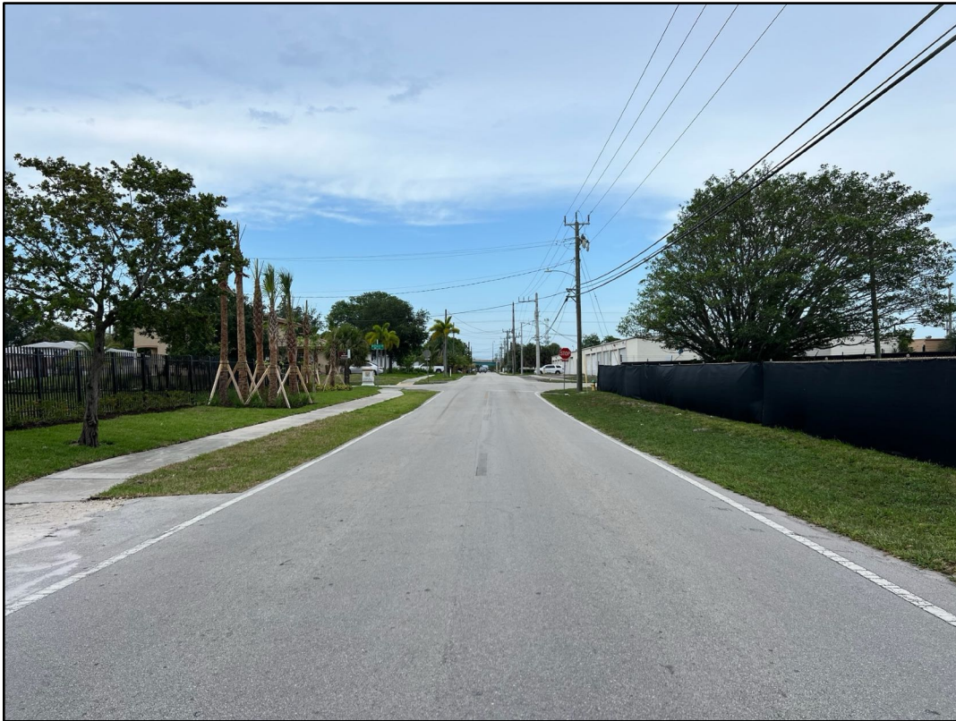
Pictured: Eller Street facing eastward. Sidewalks present on northside abutting Phase I but absent on the south for Phase II.
