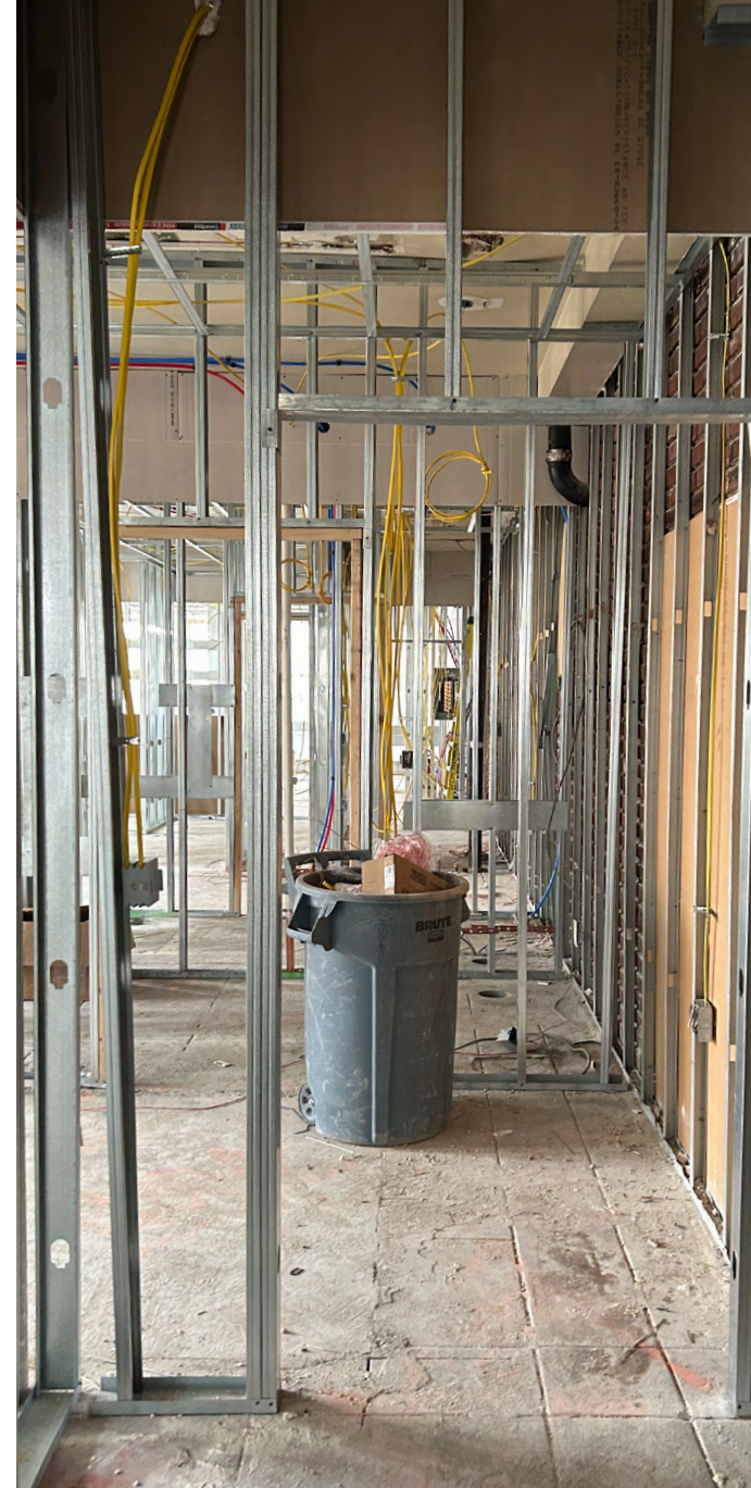
HACE's Hancock Manor apartments are undergoing significant redevelopment to improve energy efficiency and make better use of available space for tenants seeking affordable housing options.
