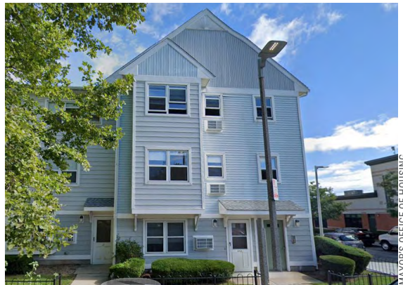
Mission Main served as a testing ground for DER measures that will be rolled out in additional buildings.
