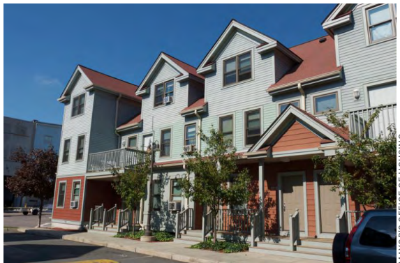
Brian J. Honan Apartments updated all systems to electric across all housing units.
