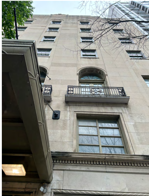
The Mid City Apartments on Chestnut Street provide critical housing opportunities to individuals who have recently experienced homelessness.
