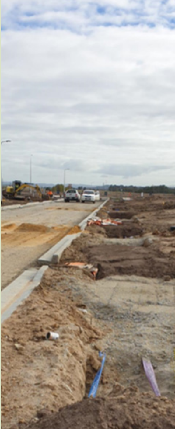
Figure 8 - Modified topsoil backfilled in tree growth zones between driveway cross overs.
