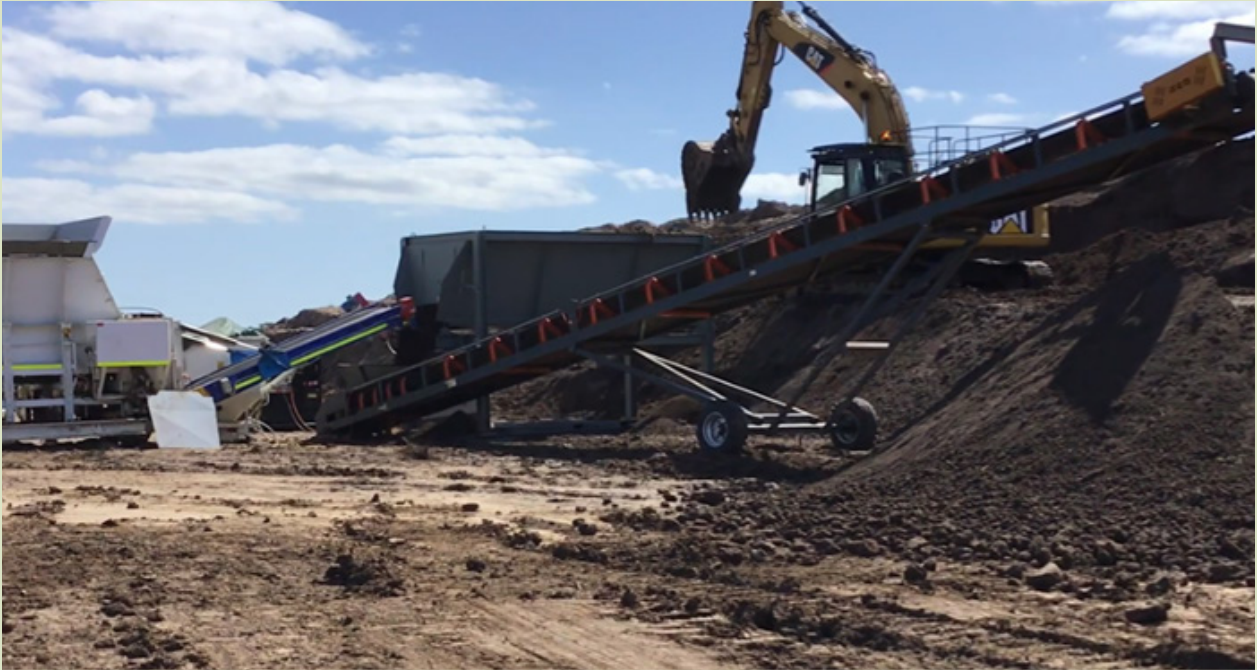
Figure 7 - Site won topsoil being ameliorated to Soil Scientist.
