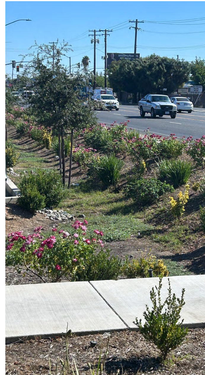
This green infrastructure is using planted materials to help absorb the water that drains from the roadway and the nearby surface parking lot.
